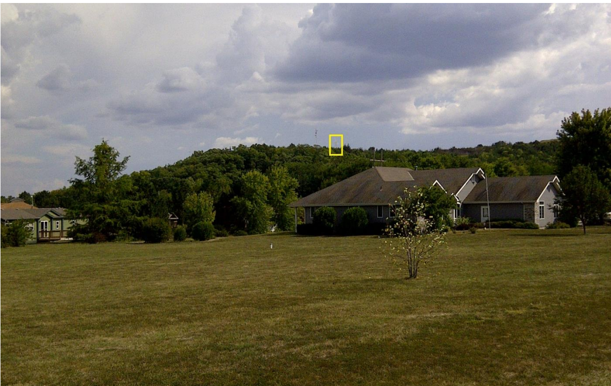
6: Southeast view of turbine and communications tower from Bent Tree Drive at US-24.
