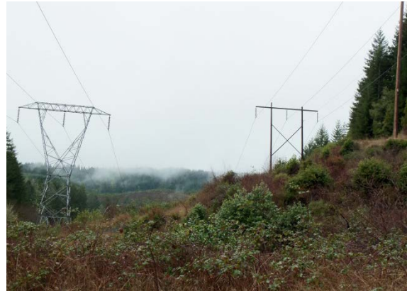
Figure 2-2. Photos of existing lattice-steel tower and wood-pole structures
