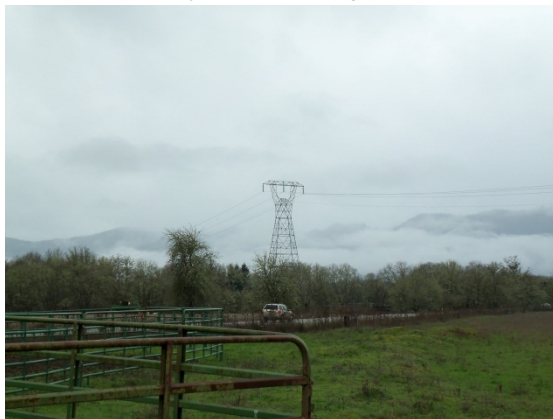
View 5: View from Tyee Road, looking southwest.
