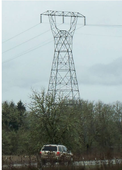
Existing transmission line Line Mile 92—two parallel lines location; BPA's Reston-Fairview 230-kV lattice-steel tower pictured on left
