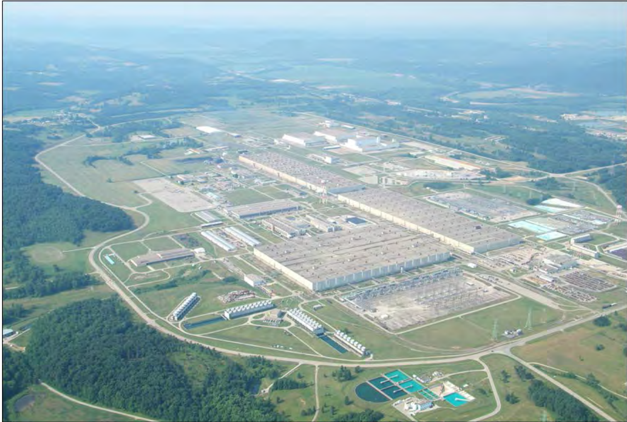
Figure 2. Aerial View of PORTS (circa early 2000s)
