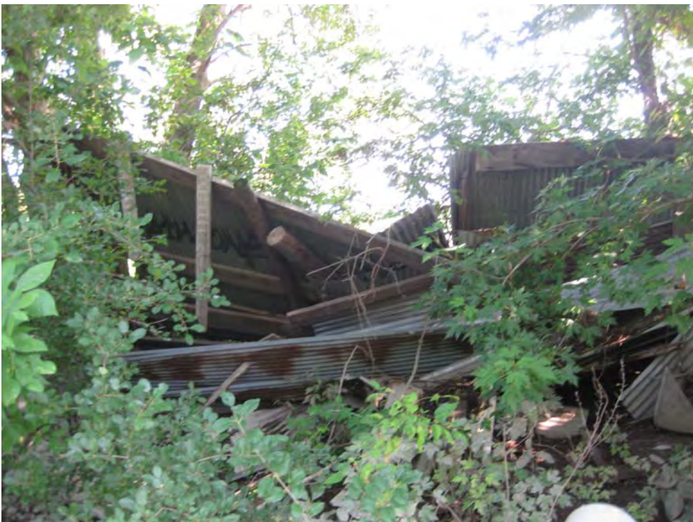
View to north. Demolished structure.
