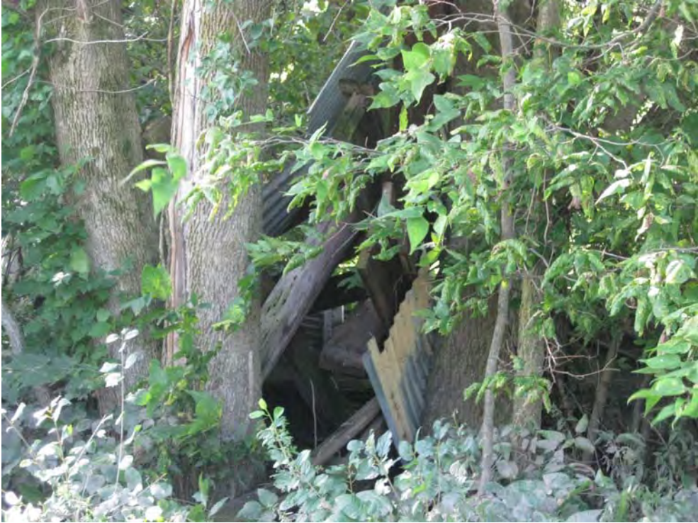
View to south. Demolished structure.
