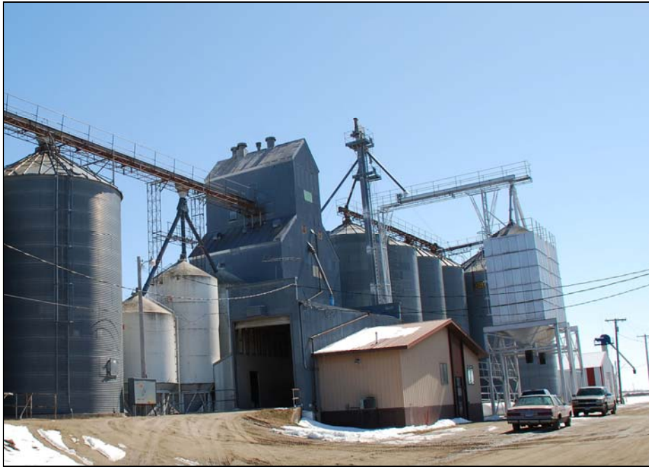
FIGURE 36. WAUBUN ELEVATOR COMPANY COMPLEX (MH-WBC-093), FACING SOUTHEAST
