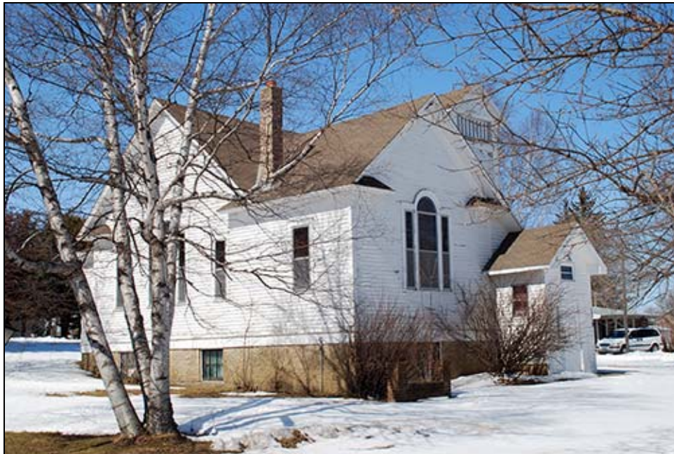
FIGURE 32. WAUBUN CONGREGATIONAL CHURCH / UNITED CHURCH OF CHRIST (MH-WBC-074), FACING NORTHWEST
