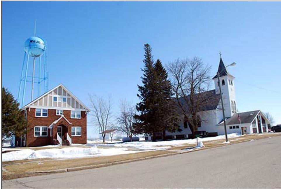
FIGURE 26. ST. ANN'S RECTORY AND CATHOLIC CHURCH (MH-WBC-004), FACING SOUTHEAST
