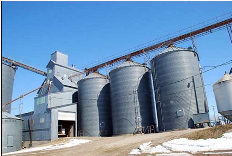
FIGURE 35. WAUBUN ELEVATOR COMPANY COMPLEX (MH-WBC-093), FACING NORTHEAST
