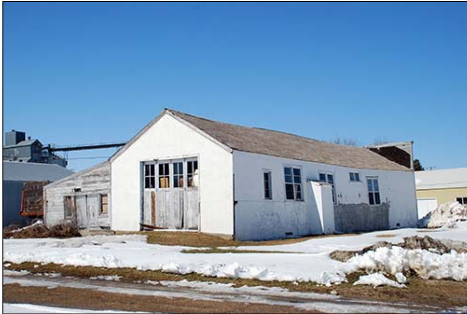
FIGURE 9. GOLDEN RULE STORE (MH-WBC-078), FACING NORTHWEST
