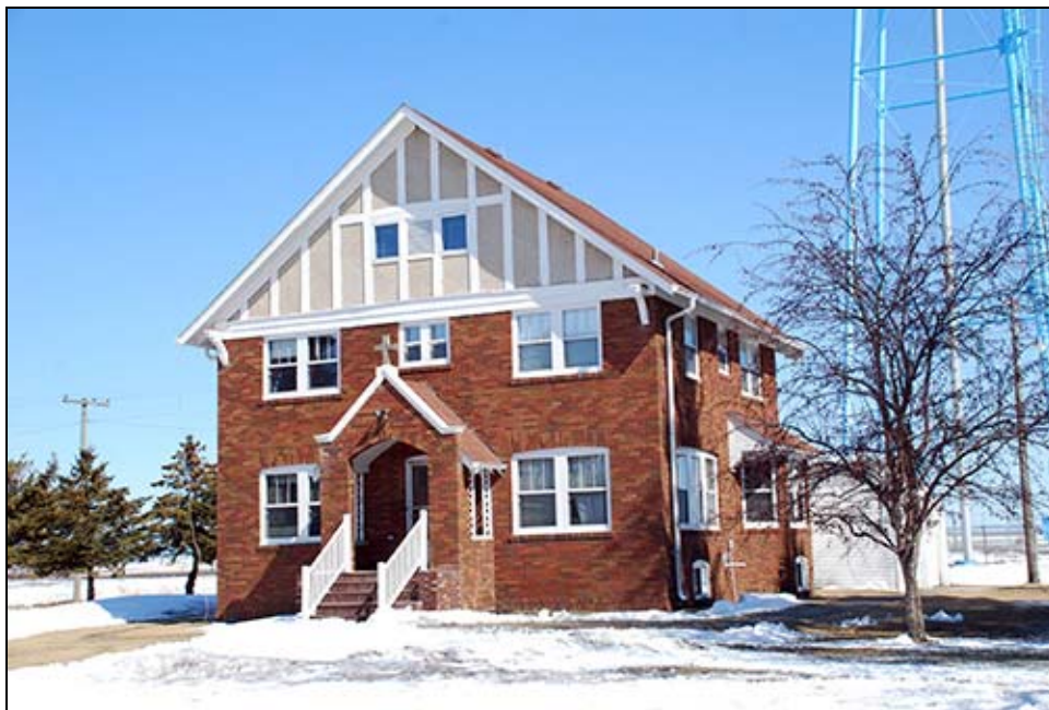
FIGURE 29. ST. ANN'S RECTORY (MH-WBC-004), FACING NORTHEAST
