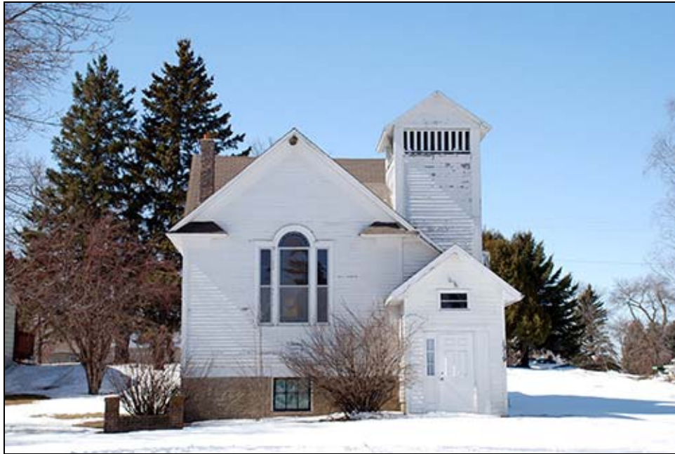
FIGURE 31. WAUBUN CONGREGATIONAL CHURCH / UNITED CHURCH OF CHRIST (MH-WBC-074), FACING WEST
