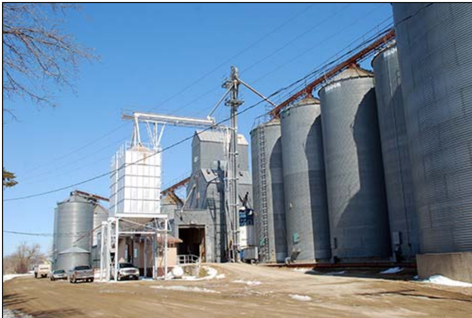
FIGURE 37. WAUBUN ELEVATOR COMPANY COMPLEX (MH-WBC-093), FACING NORTH
