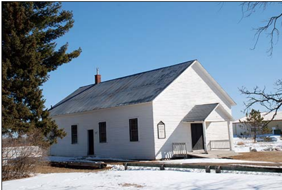
FIGURE 20. KATERI TEKAKWITHA HALL (BK-PNP-001), FACING NORTHEAST
