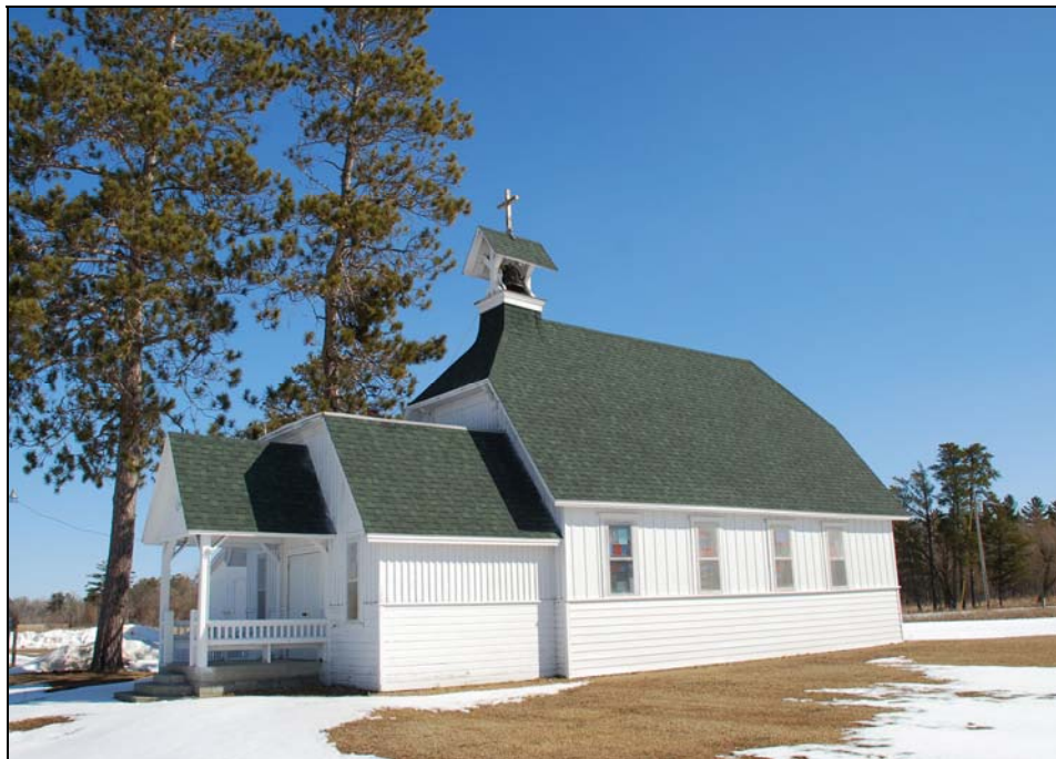
FIGURE 24. BRECK MEMORIAL EPISCOPAL CHURCH (BK-PNP-007), FACING NORTHEAST
