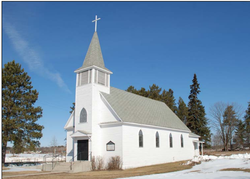
FIGURE 16. ST. THEODORE'S CATHOLIC CHURCH (BK-PNP-001), FACING NORTHWEST
