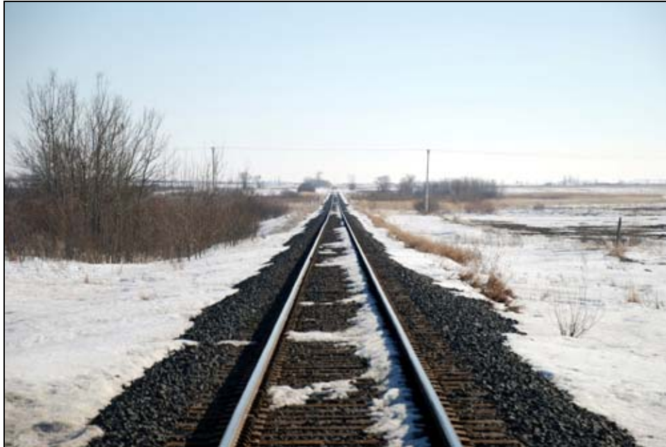
FIGURE 7. MStP&SSM / SOO LINE / CP RAILWAY (MH-PGR-002), FACING SOUTH
