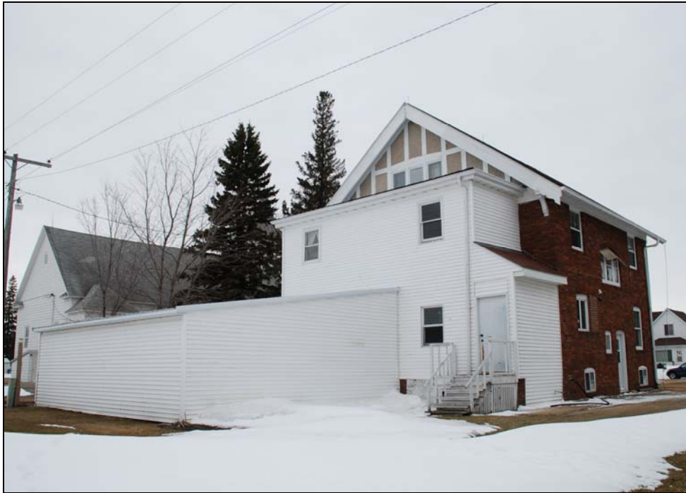
FIGURE 30. ST. ANN'S RECTORY (MH-WBC-004), FACING SOUTHWEST
