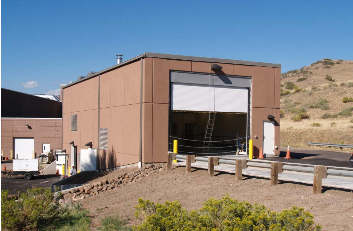
Figure 2-3. View of the east side of the RFHP at the unloading area for woodchips. Open bay door leads to the fuel pit. Proposed silo would be located on the asphalt area to the left and below the building.
