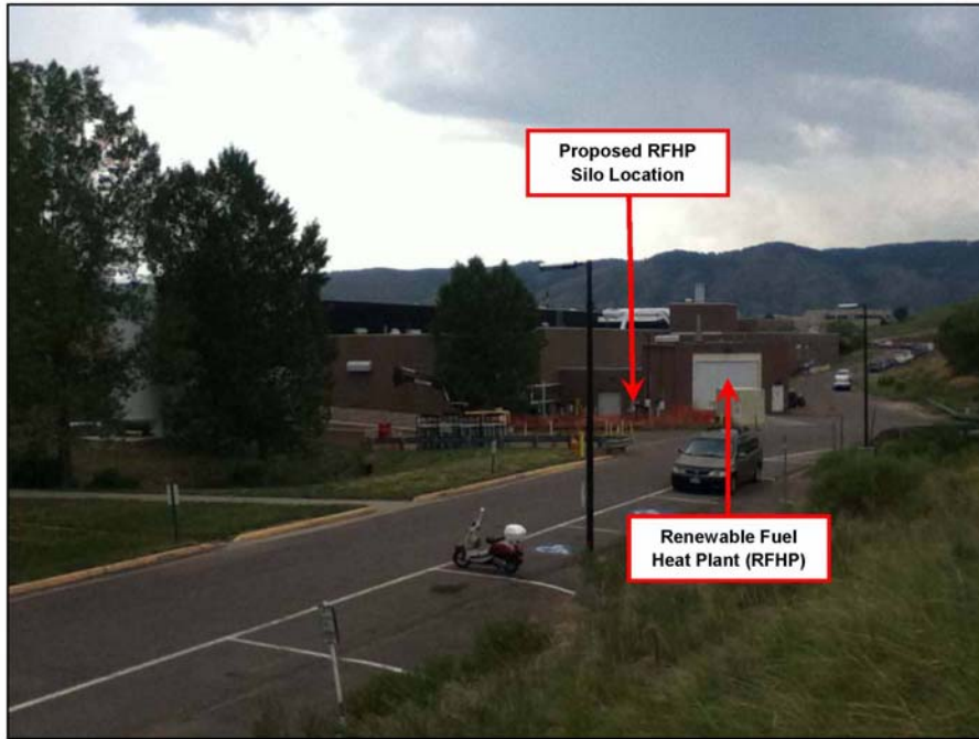
Photo 1. View from Ammunition Igloo to the southwest toward the RFHP.
