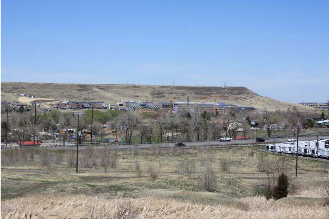
Figure 3-4. Current view of the STM site in April 2011 as seen from the U.S. Highway 6 exit ramp westbound to I-70.
