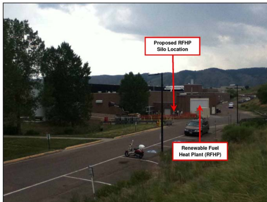
Photo 4. View from Ammunition Igloo to the southwest toward the RFHP.
