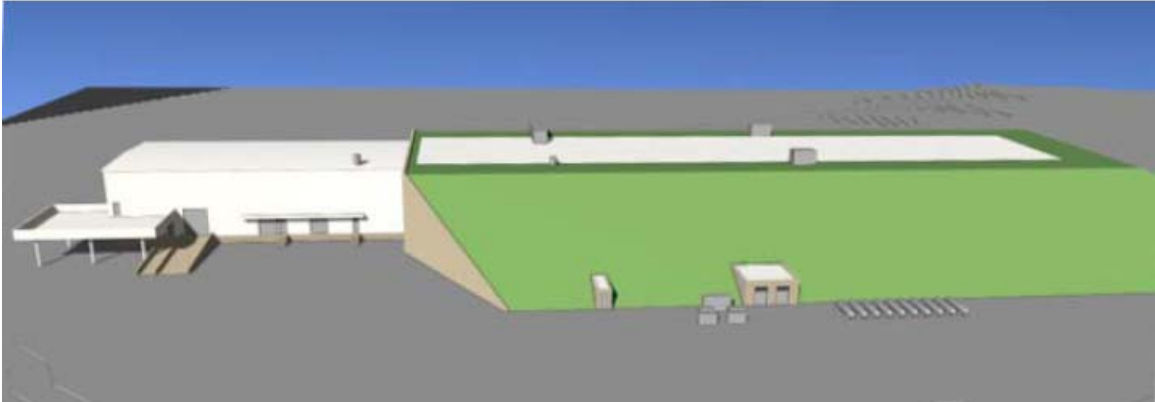
Figure 3.9: A perspective view of the proposed NO \nu A Far Detector building looking east. The bermed area (green) is composed of granite spoils from the excavation. The detector area would be on the right hand side with a module assembly area to its left. A loading dock service area is located to the left of the Assembly Area with recessed and drive-in truck bays. A scintillator tanker handling area is shown on the far left with adjacent bays for four tanker trucks.
