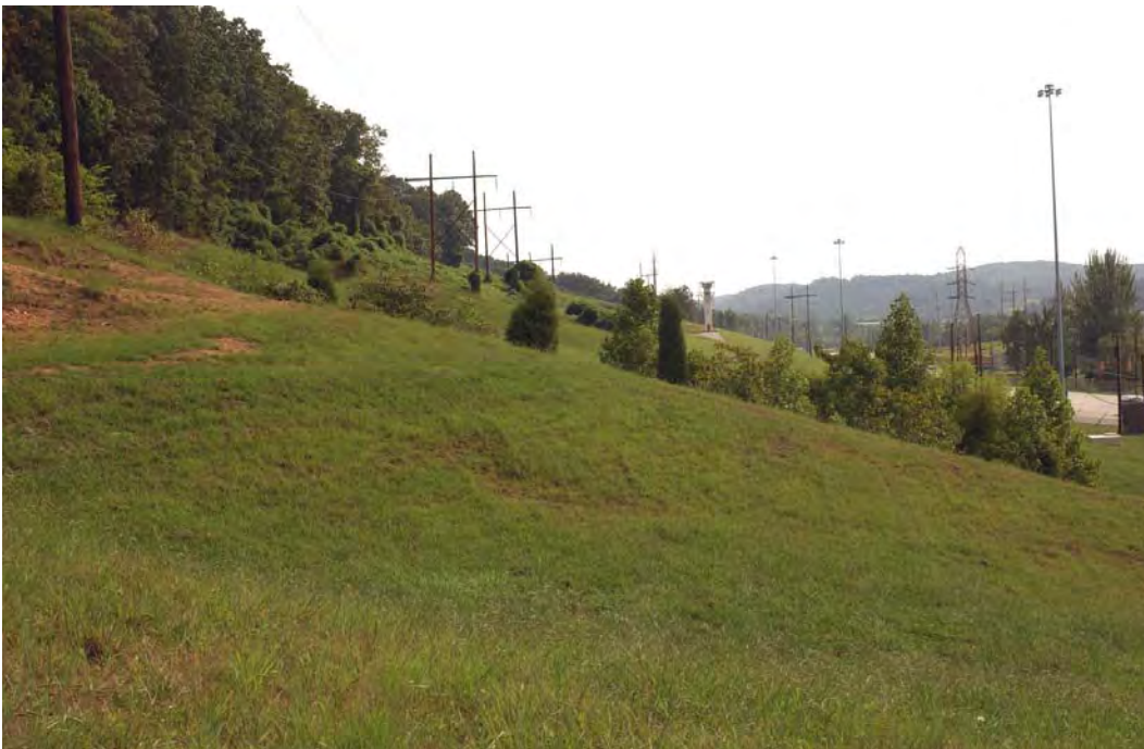
Plate 6. General View East of Force Main From Terminus of Project.
