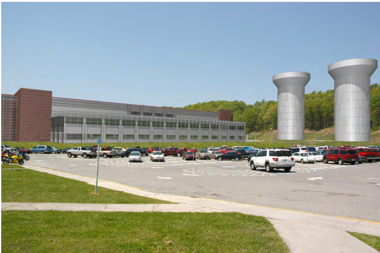
Figure 4.13-1. Visual Rendering of Elevated Water Tanks at Y-12 – Looking Northwest.
