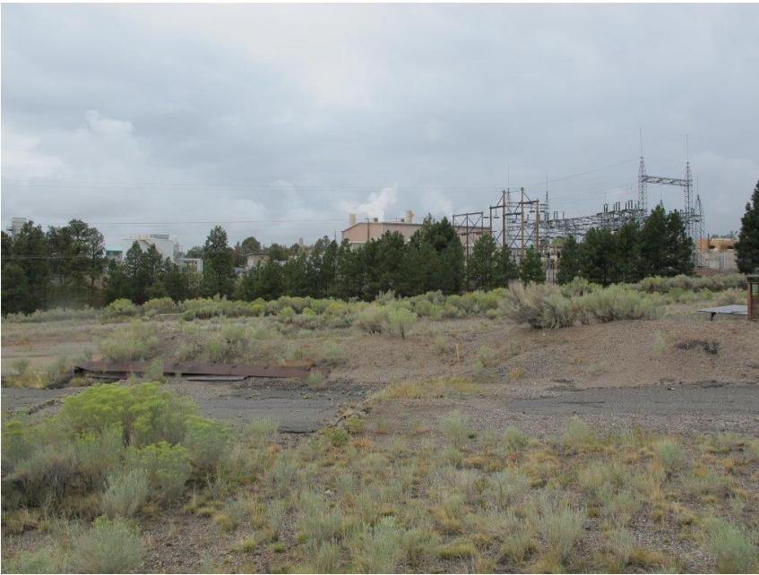
North Side of Proposed Substation Facing Southwest. Existing Substation is in the background.
