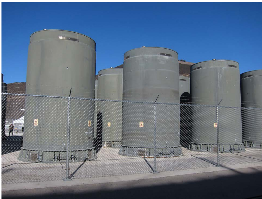
Figure 1. Holtec HI-STORM dry cask storage systems at Diablo Canyon.
