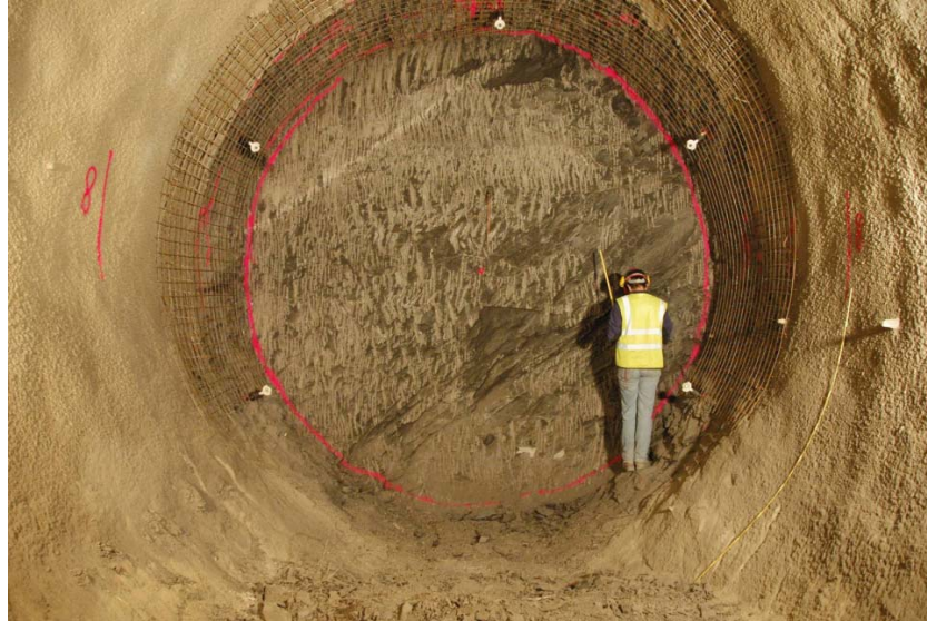
Figure 4-5. View of FE tunnel face from the FE niche showing beddings dipping 45^\circ (Viotor, 2012).
