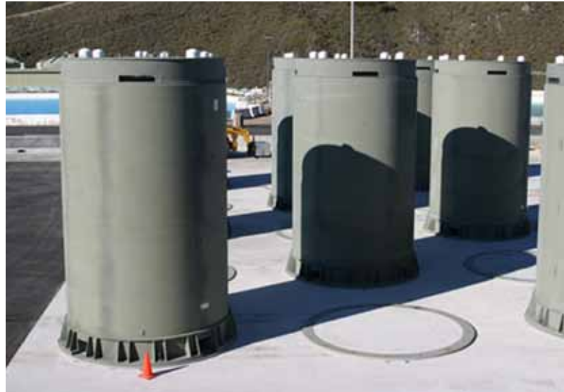
Until a permanent repository is available, UNF continues to be stored in dry casks and spent fuel pools at geographically distributed utility sites.
