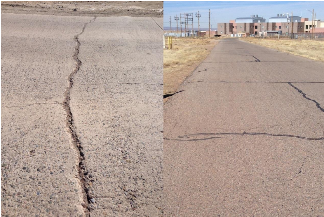
Figure 4.11 Area III road (rough asphalt), Segments 1 and 5.
