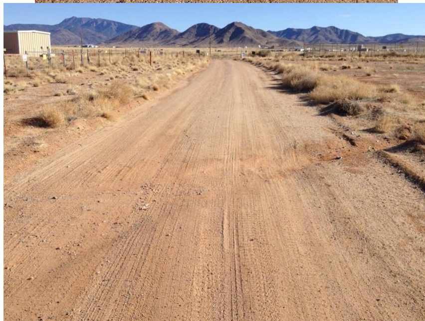
Figure 4.14 Dirt road into Building 6922 (southwest, top, and northeast, bottom), Area III, end of Segment 5. The trough shown is over 8 inches deep. The truck traveled directly over the deepest portion of the trough.
