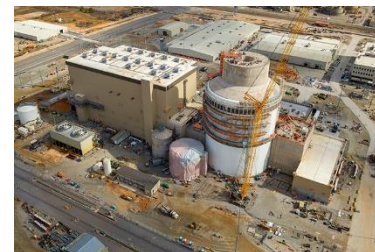
Vogtle Unit 3 (Courtesy of Georgia Power/ Southern Company, April 2021)
