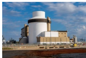
Vogtle Unit 3 (Courtesy of Georgia Power/ Southern Company, October 2022)
