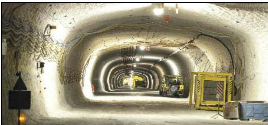
Figure 4.2-1 View of one of the underground tunnels at Gorleben at the 840 m level (BMW 2008).
