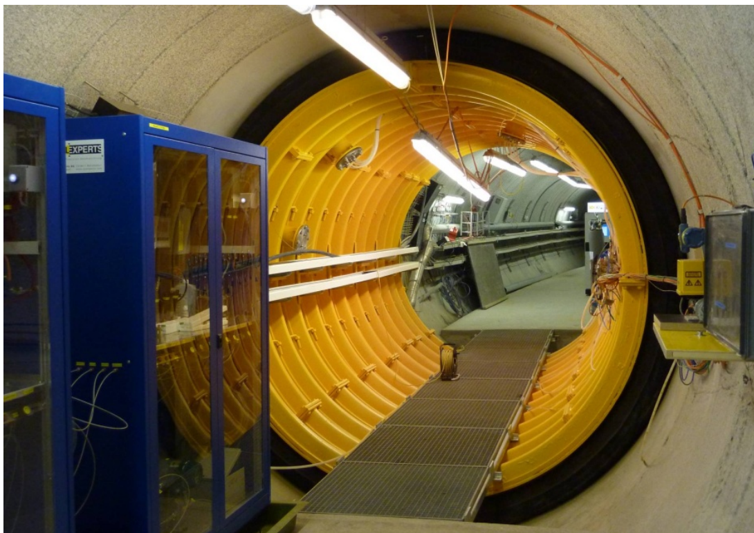
Figure 3.3-3 CFM field test bed at Grimsel Test Site: Tunnel packer system used to isolate the shear zone ( http://www.grimsel.com/gts-phase-vi/cfm-section/cfm-site-preparation ). Small disks with tubing issuing from them (inside yellow packer) are “surface packers” that seal the tunnel wall and collect water from inflow points. Tunnel diameter is 3.5 meters.
