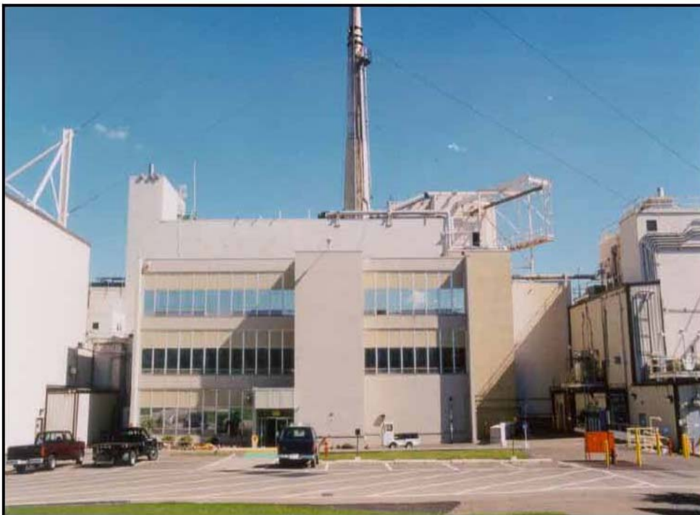
Figure 3-14. West Side of the Process Building. (The building with windows is actually the Plant Office Building. The plant part of the Process Building is behind the Office Building)
