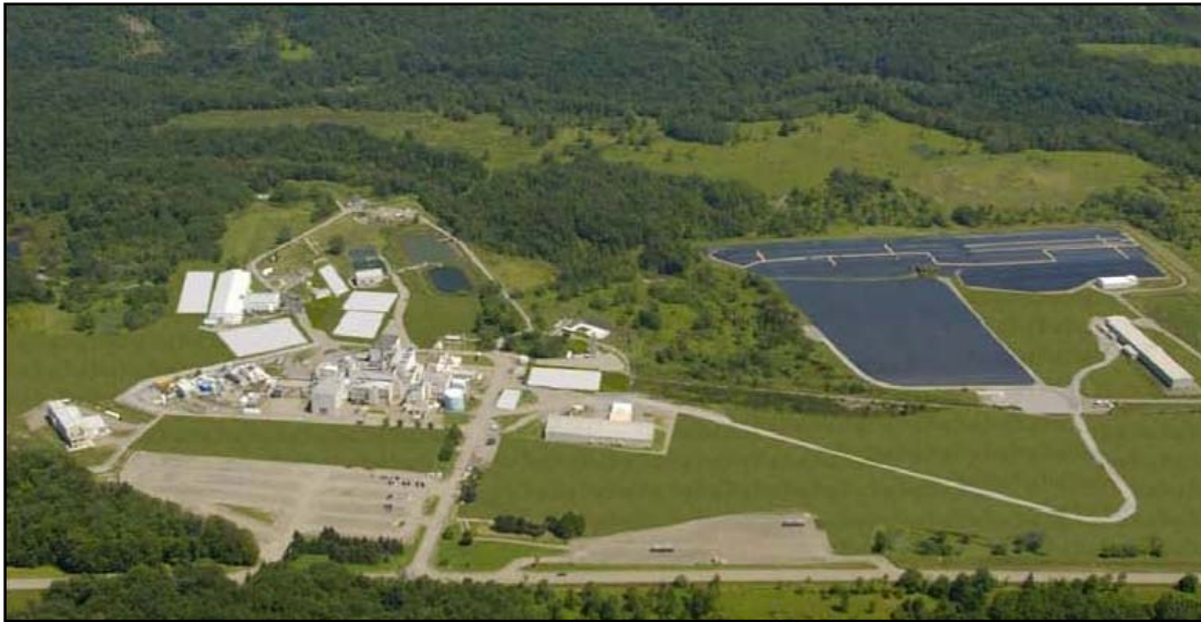
Figure 1-7. The WVDP in the Interim End State
