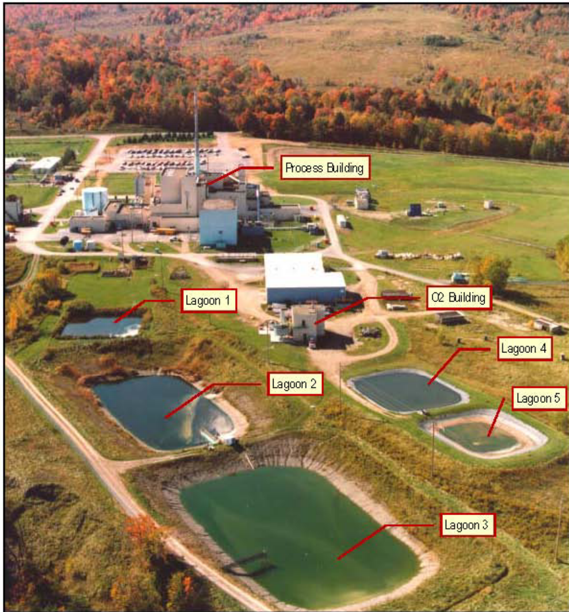
Figure 3-25. The Low-Level Waste Treatment Facility. (This photo shows the site in 1982, looking toward the southwest.)
