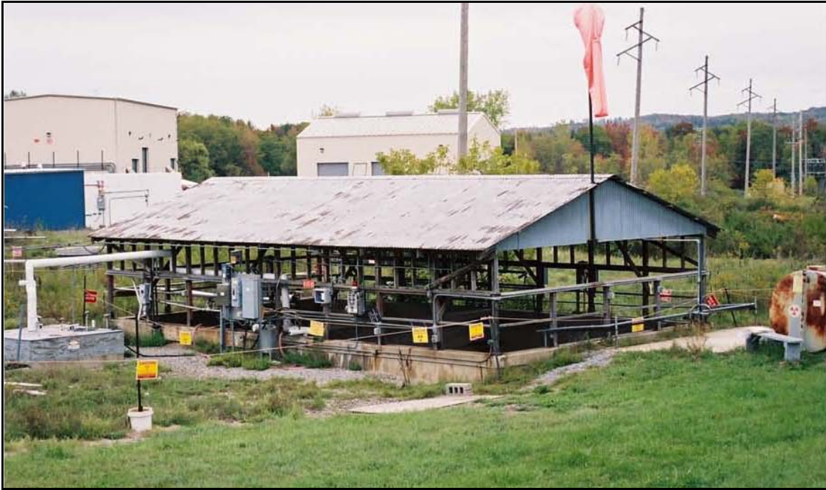
Figure 3-28. The New Interceptors. (These are twin stainless-steel lined concrete holding tanks.)
