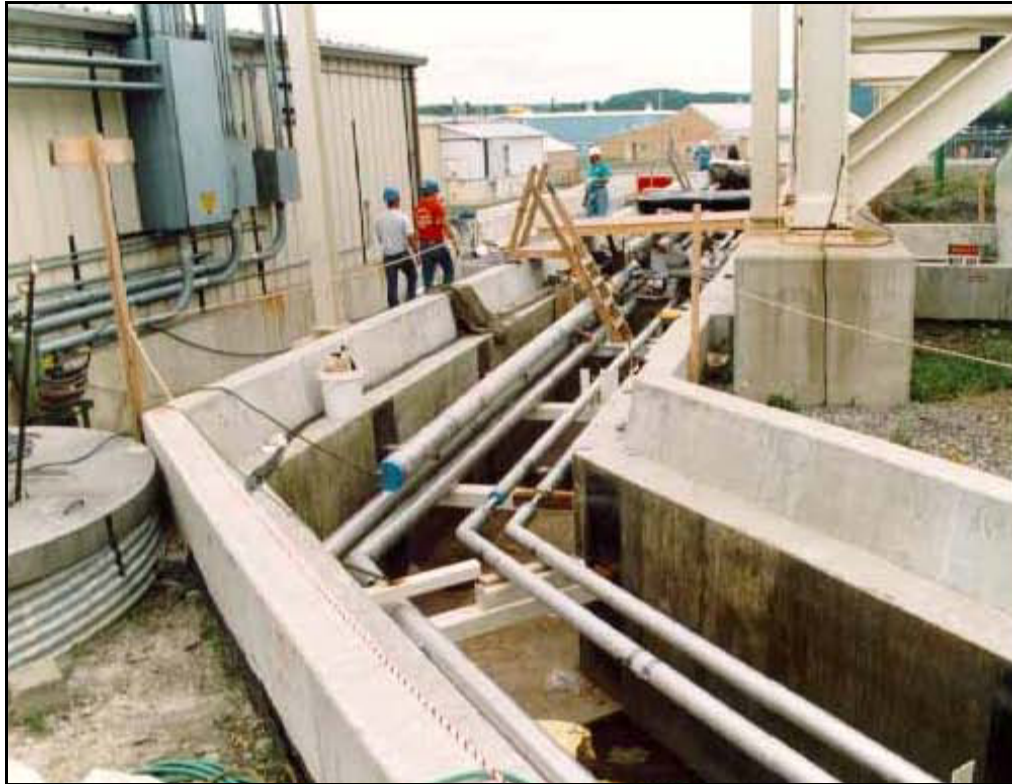
Figure 3-33. HLW Transfer Trench Under Construction
