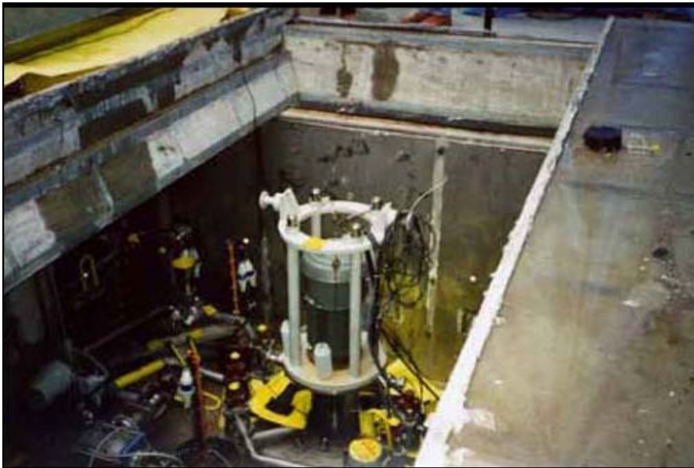
Figure 3-34. Typical HLW Pump Pit
