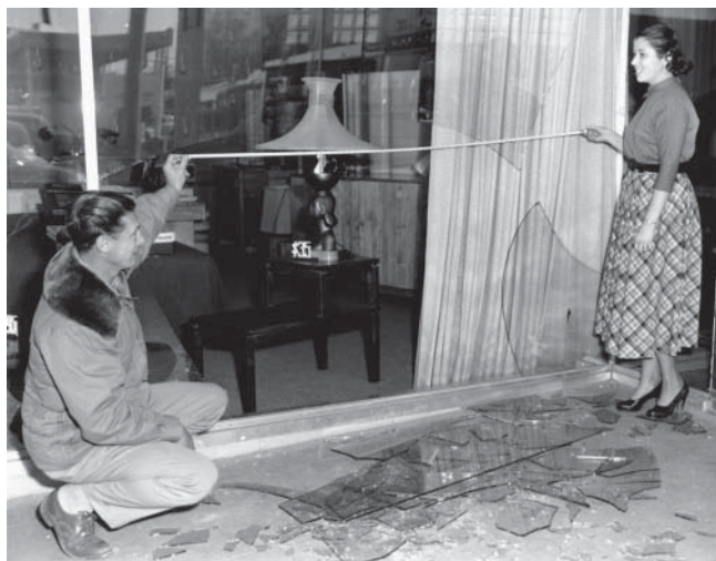
Broken plate glass window in downtown Las Vegas from the Baker-Two shot. Source: AP/Wide World Photos.
