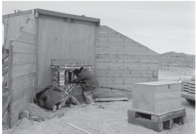
Putting detonators in place at zero shack. Source: Los Alamos National Laboratory.
