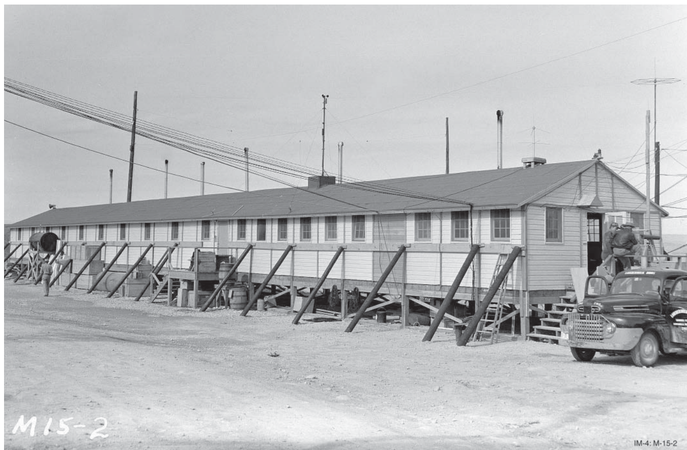
South side of the control point building. Entrance to the control room is at right. Men on porch are looking north toward ground zero. Note braces shoring up the building. Source: Los Alamos National Laboratory.
