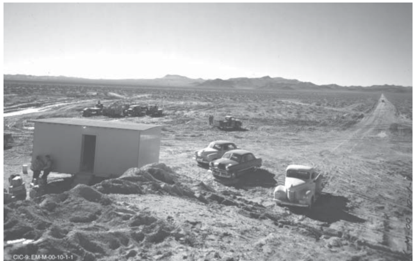
Construction near ground zero. Source: Los Alamos National Laboratory.
