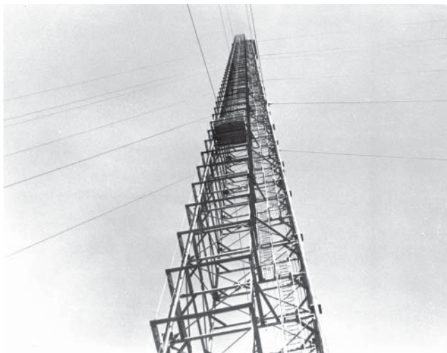
The 700-foot tower, top, at the north end of Yucca Flat for the Smoky shot. The top of the tower, bottom, viewed from its base. About half way up is the elevator featuring an electro-magnetic system of control that eliminates the need for trailing cable below the elevator. Source: DOE, NNSA-Nevada Site Office.
