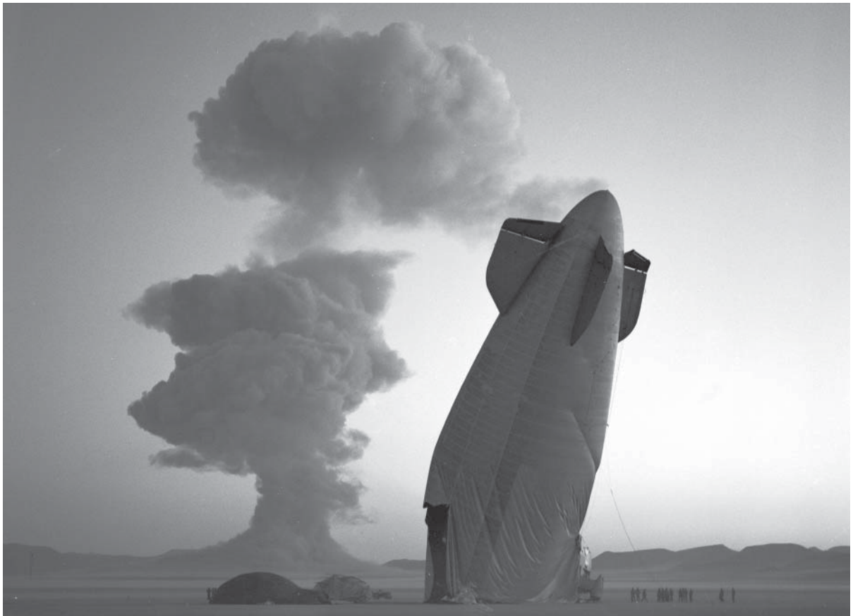
Navy air ship, ZSG-1, top, tied up at mooring platform at Yucca Flat, having just arrived from Lakehurst (NJ) Naval Air Station. The tail, or after section, bottom, of a Navy blimp is shown with the Stokes shot cloud in background. Blimp was in temporary free flight in excess of five miles from ground zero when collapsed by the shock wave from the blast. The airship was unmanned. On ground to the left are remains of the forward section. Source: DOE, NNSA-Nevada Site Office.
