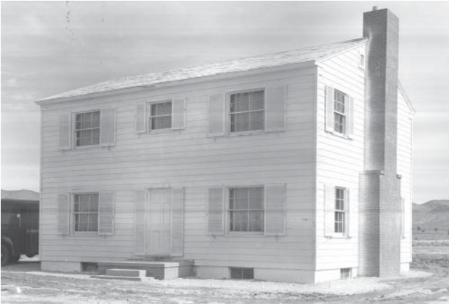
One of the two frame houses built 3,500 and 7,500 feet from ground zero. Source: DOE, NNSA-Nevada Site Office.
