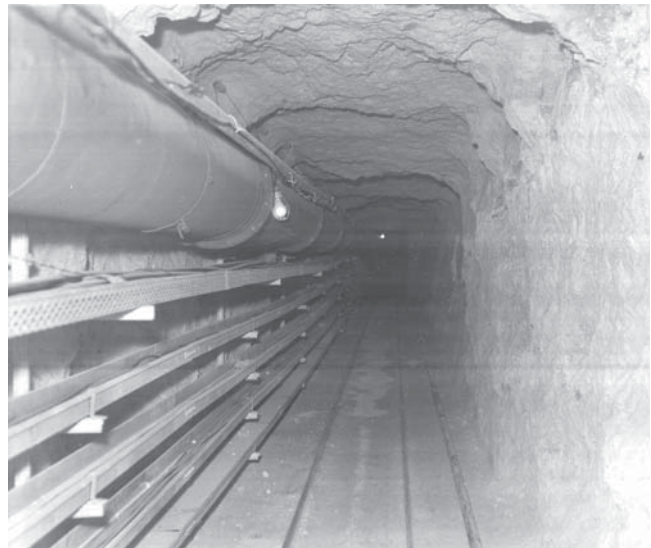
Post-shot view of a portion of the Rainier tunnel not far from its entrance with ventilation duct (large pipe) and diagnostics cable racks at left. Source: DOE, NNSA-Nevada Site Office.
