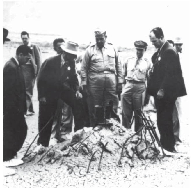
Remains of Trinity tower footings. Oppenheimer and Groves at center. Source: Department of Energy.
