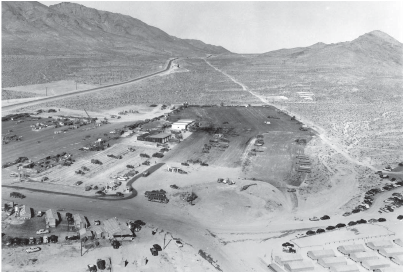
Camp Mercury during construction. Source: DOE, NNSA-Nevada Site Office.
