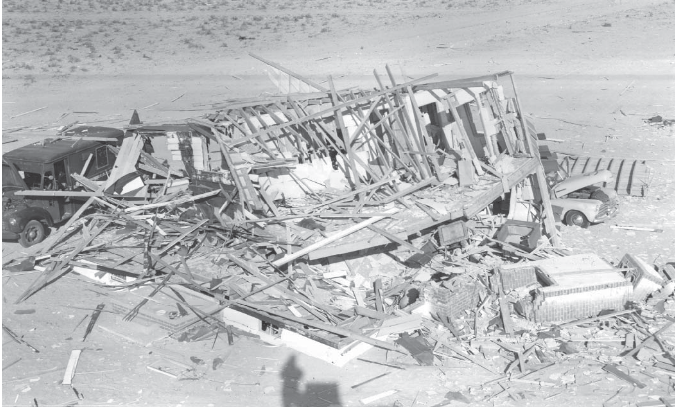
Demolished wooden house and two vehicles. Source: DOE, NNSA-Nevada Site Office.
