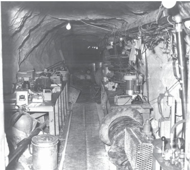
Diagnostic instruments in the diagnostics room of the Rainier tunnel. Source: DOE, NNSA-Nevada Site Office.
