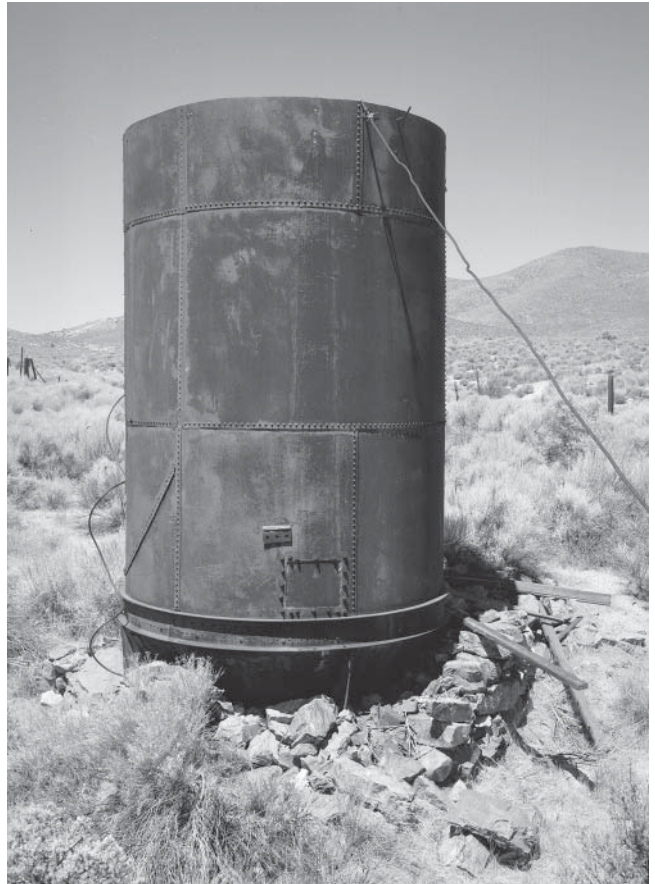
Tippipah Spring, top, with water storage tanks made from a boiler. Source: DOE, NNSA-Nevada Site Office.
