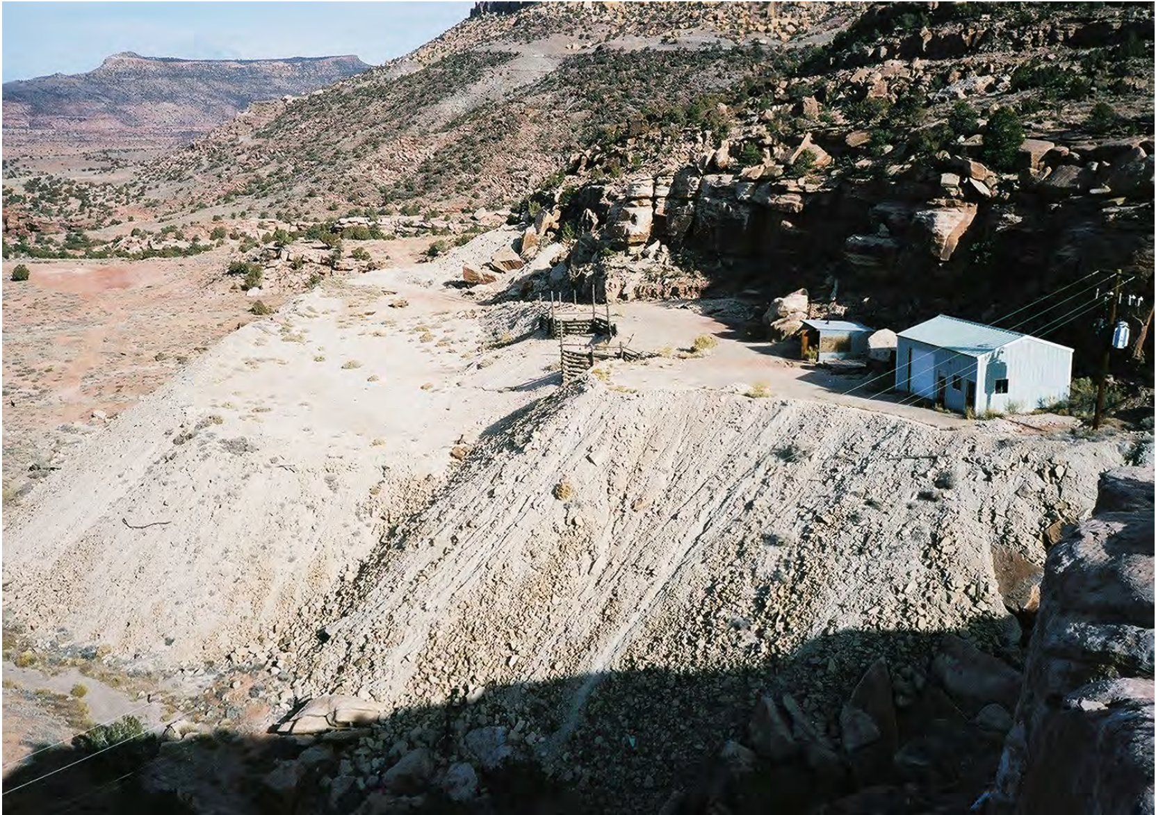
FIGURE 2.1-4 Photograph of Former Mine Plant Surface Configuration at Lease Tract 13A
