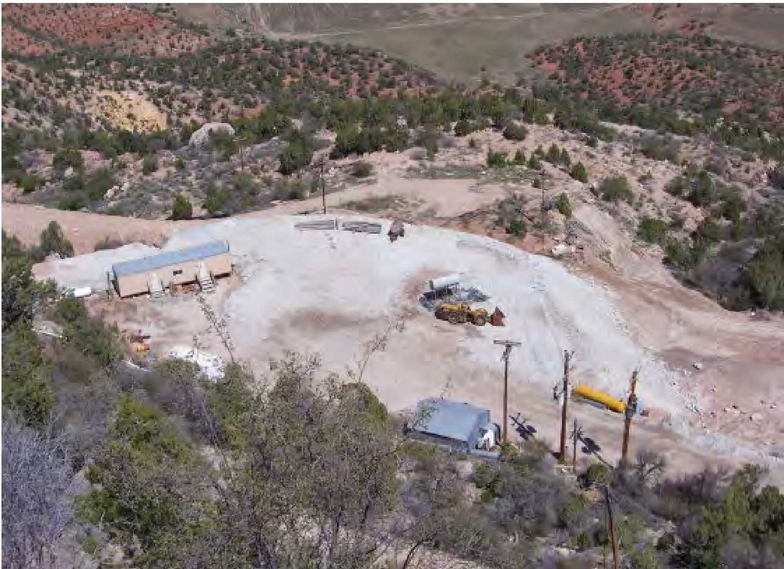
FIGURE 2.1-3 Photograph of Mine Plant Surface Configuration at Lease Tract 8
