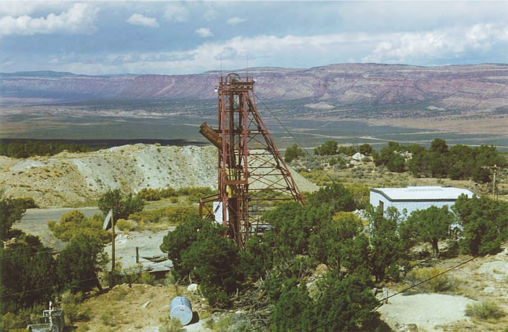
1 2 FIGURE 2.1-1 Photograph of Mine Plant Surface Configuration at Lease Tract 5
