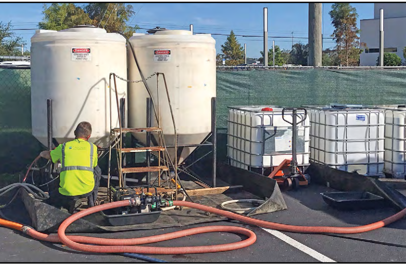
A bioinjection solution mixing station at the Pinellas County site.
