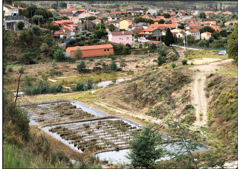
Cunha Baixa Old Mine in Portugal. Remediation technologies include active and passive wastewater treatment systems near a residential area.
