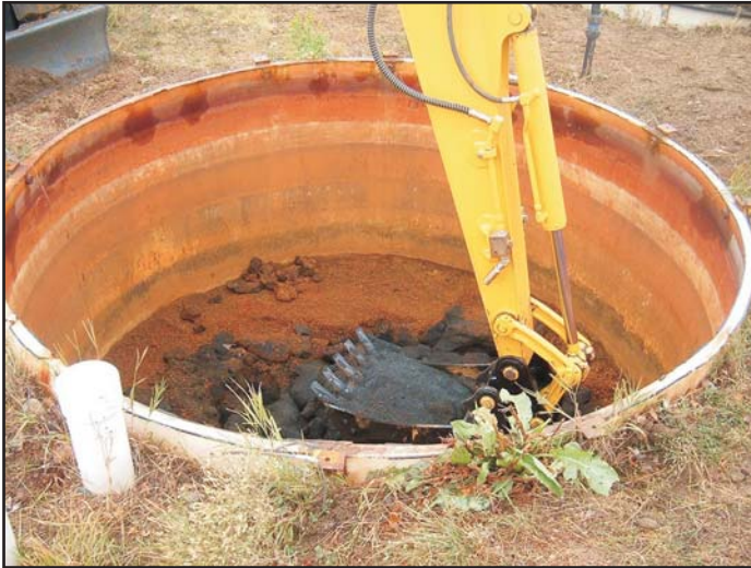
During media removal you can see the mineralized ZVI that has become crusted and turned orange, while the black ZVI in the center of the cell shows little sign of contact with water flow.
