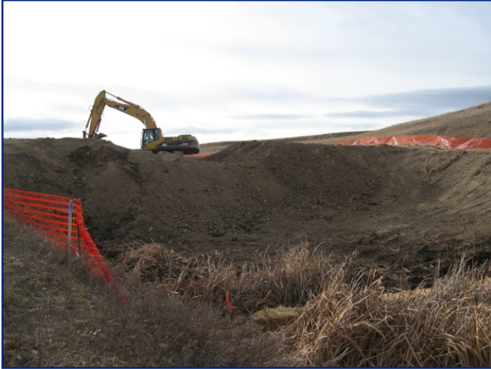
An excavator starts cutting the notch in a dam.
