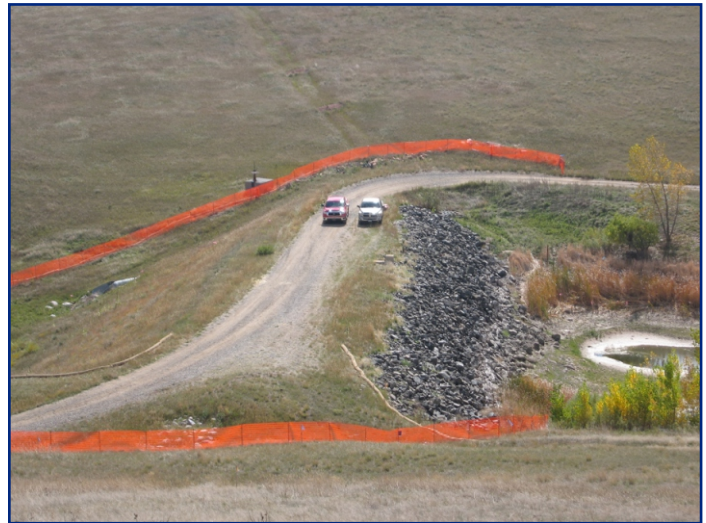
A view of the A-2 pond dam prior to breaching activities.
