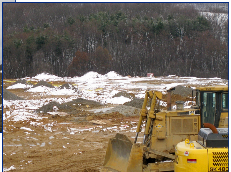
Looking past earth-moving equipment toward foundation work (caissons).
