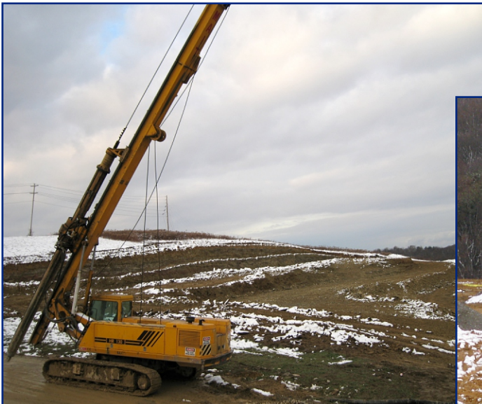
Auger in foreground of cut area on western portion of site.
