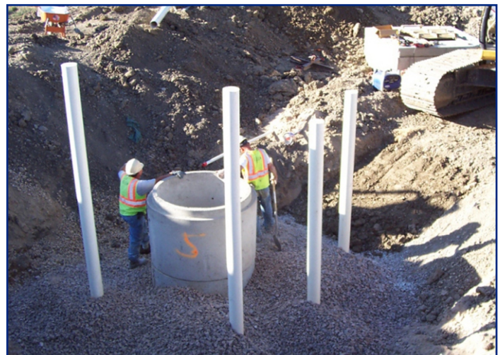
Collection sump installation at the SPPTS.
