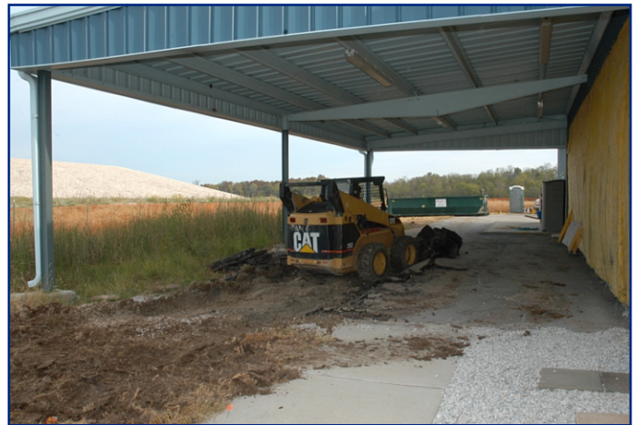
Old asphalt under the Interpretive Center canopy was removed.
