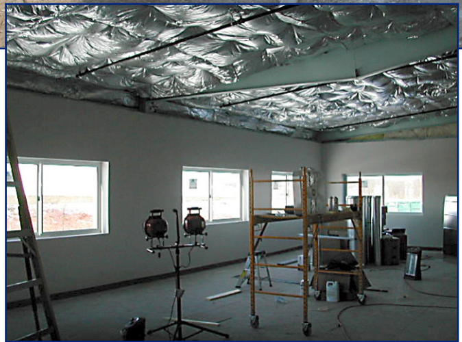
Top photo: A new concrete foundation was poured under the canopy. Bottom photo: An interior view of the new meeting room. A drop ceiling will be installed and the entire space will be freshly painted.
