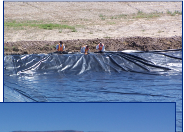
Installation of In-Cell Pond Liner.
