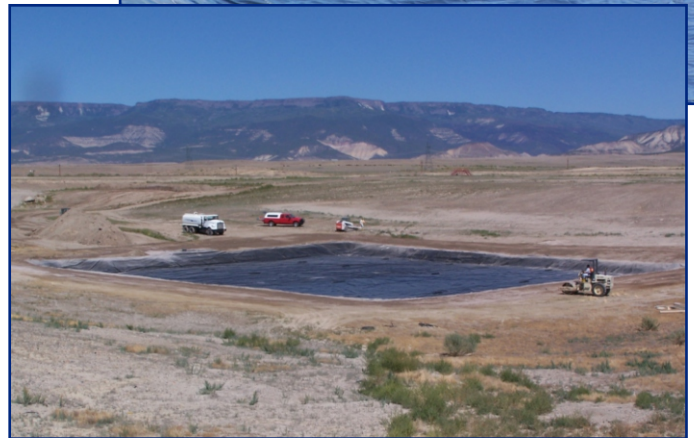
Completed Installation of In-Cell Pond Liner.
