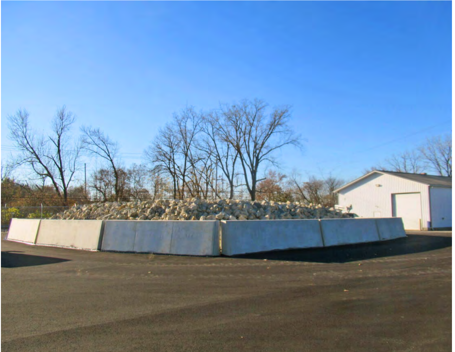
The entombment sits below grade, fully enclosed in a 10-foot-thick concrete barrier. The surface includes a vegetation barrier and loose stone cover, known as riprap, secured by heavy-duty jersey barriers. The city can use the surrounding parking lot as a laydown area.
