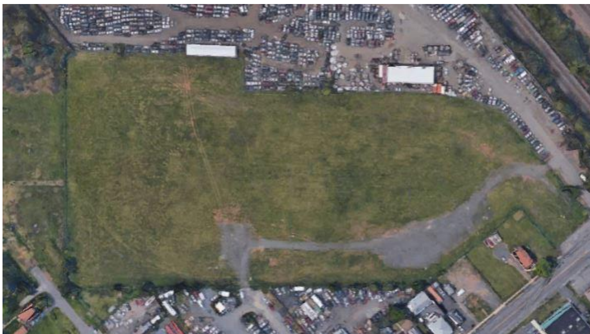
Fig. 2. Middlesex South Site Conditions 2019 with Interim Storage Piles Removed
