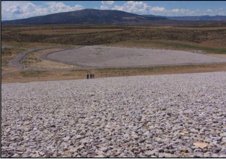
View from the Disposal Cell Looking South Toward the Ancillary Cell.
