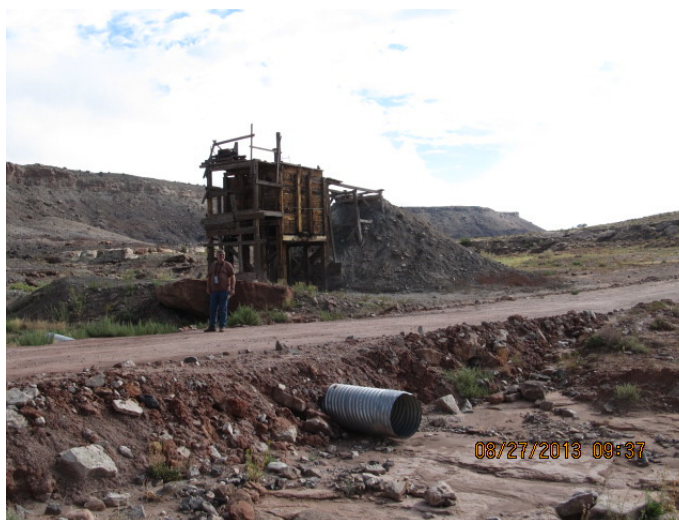
Figure 7. Load-Out Prior to Reclamation
