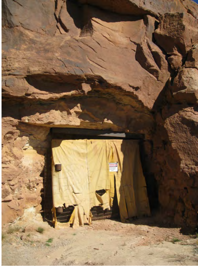
1 2 FIGURE 3.12-8 View of Entrance to Underground 3 Mine at Lease Tract 18 (The Cotter Mine entrance 4 has a locked gate to prevent unauthorized entrance 5 and is covered with fabric to control ventilation.) 6 7
