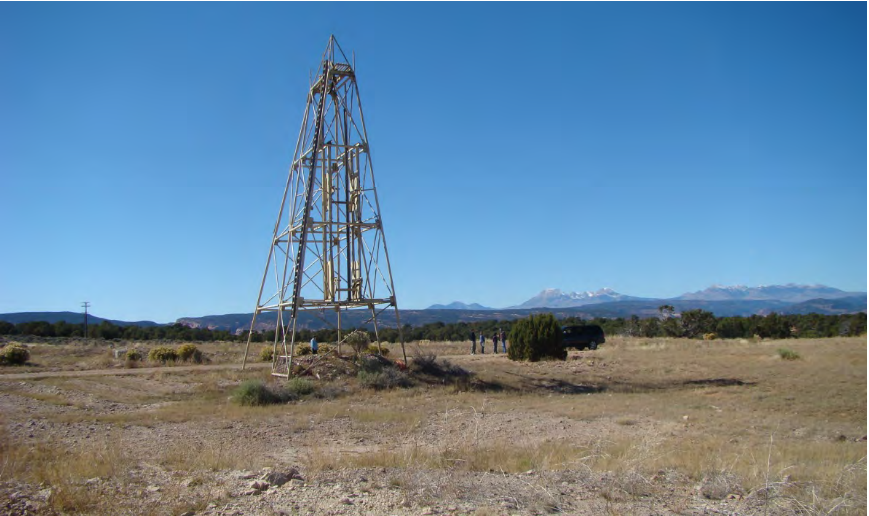
FIGURE 3.12-7 View of Lease Tract 19 Facing West (A headframe structure is located above the closed shaft of the Golden Cycle underground mine.)
