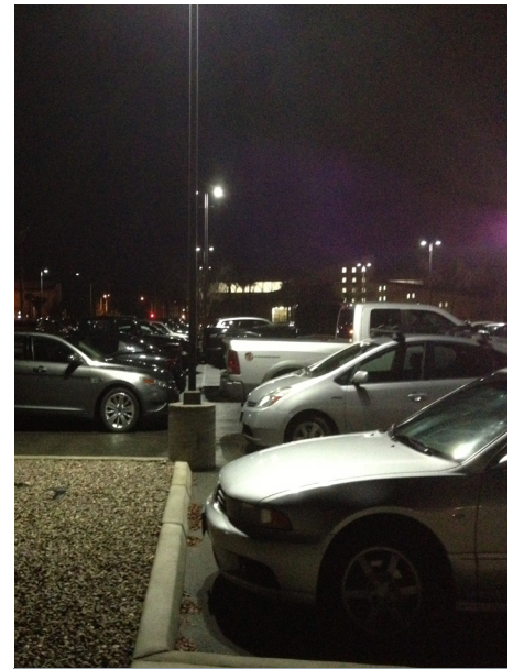
The pre-retrofit high-pressure sodium lamps produced a yellow light while the new induction lamps produce a bright white light, improving color rendering and visibility. Photo courtesy of MCBCP.
