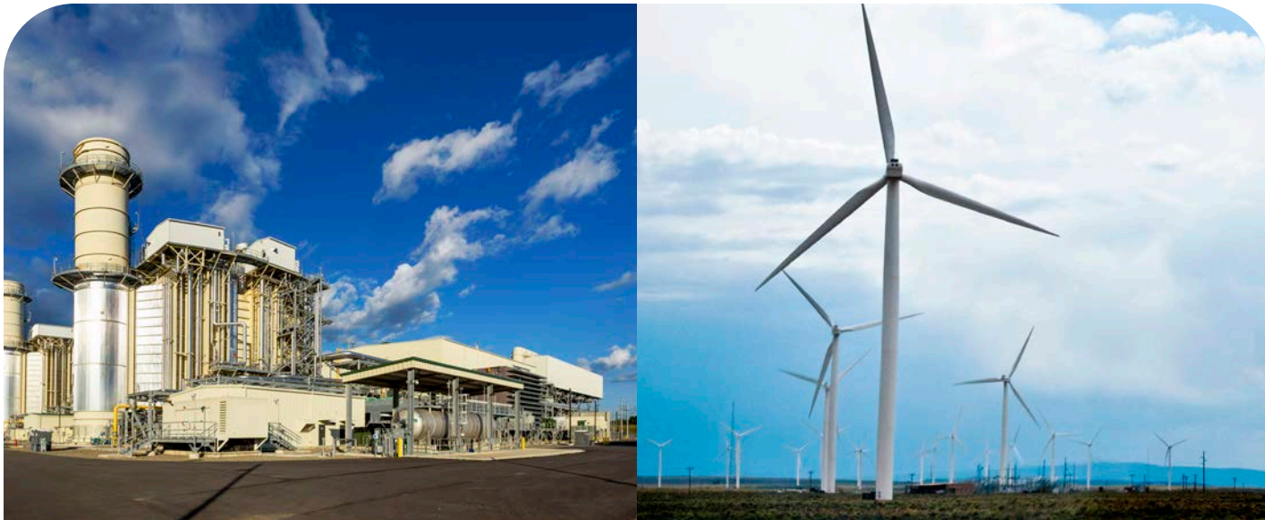
Flexible natural gas-fired power generation plants (left) help ensure that wind power remains reliable (right).
