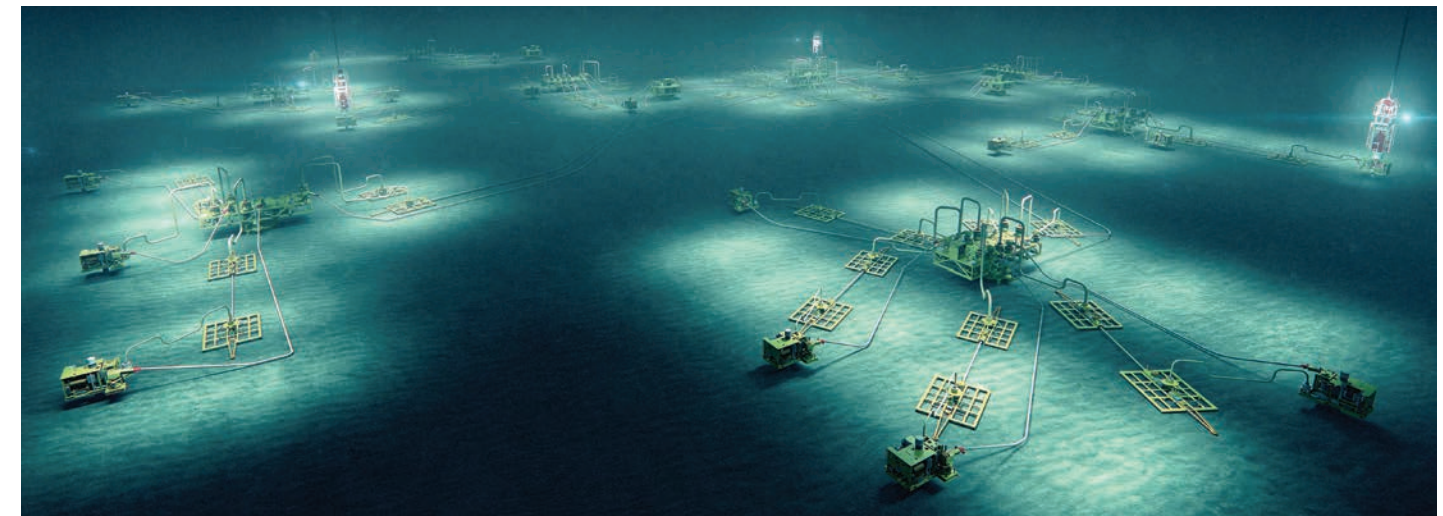
Artist's depiction of a subsea factory meant to replace floating or fixed production facilities. Individual wells are connected to centralized produced oil processing units. Injected CO 2 is removed from the produced oil and re-injected, all on the seafloor.
