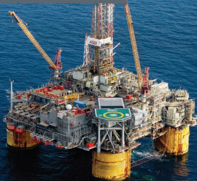
Shell's Auger tension leg platform in Garden Banks Block 426 is tethered to the seafloor in 2,360 feet of water.
