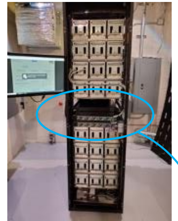
Server rack containing Natron batteries
