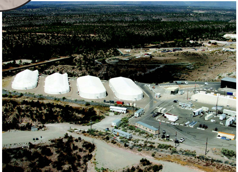
Waste Storage Domes at Area G
