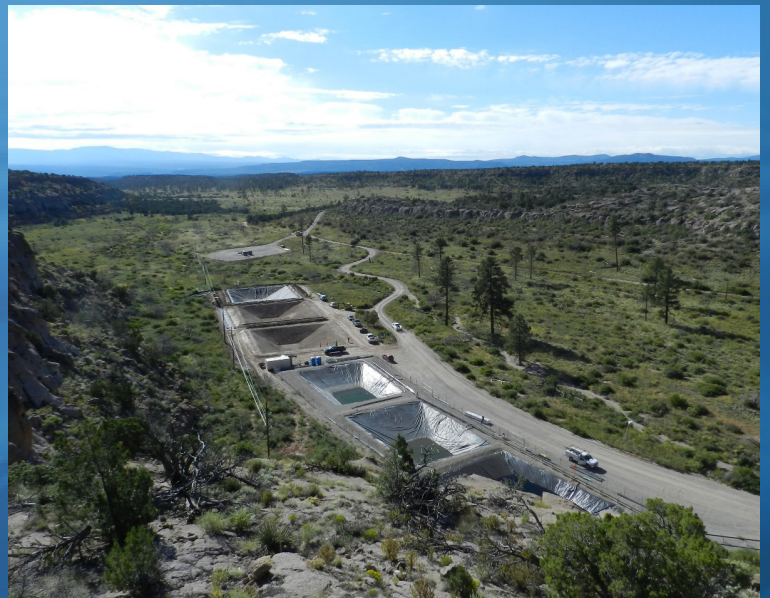
Storage basins in Mortandad Canyon store treated groundwater prior to land application.
