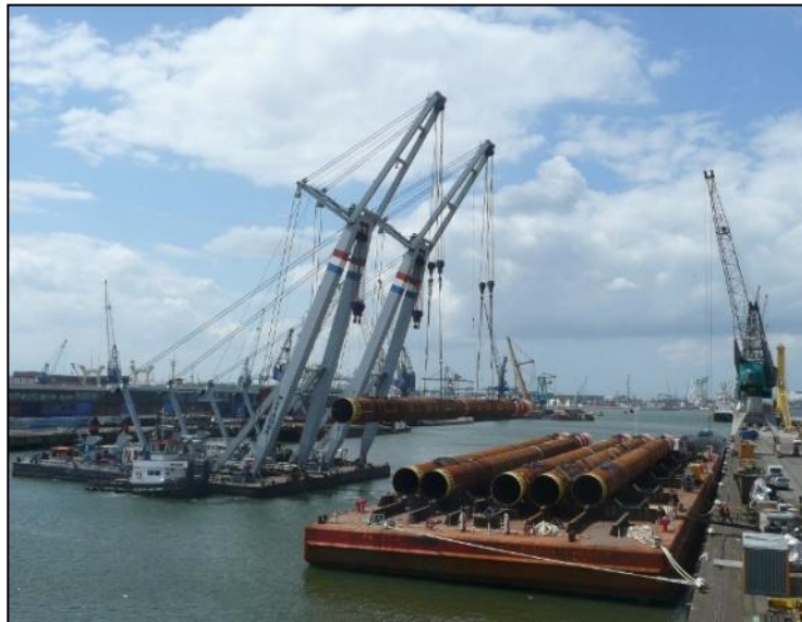
Figure 3-5: Monopiles being loaded onto a Deck Barge by Shearleg Cranes
