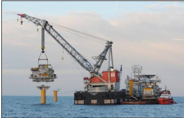
Figure 3-11: Substation Topside Installation (heavy-lift crane vessel)
