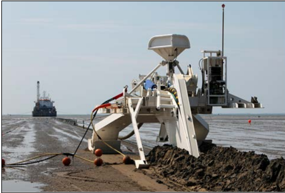
Figure 3-13: Subsea Cable Plow Burying Cable at Shore
