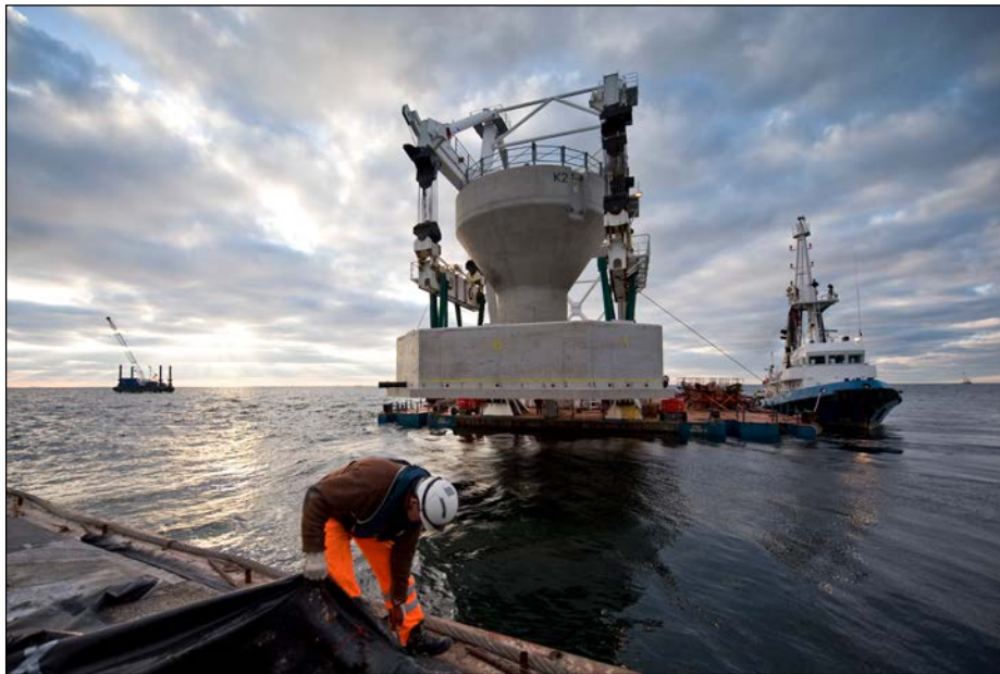
Figure 5-24: Eide 5 Heavy-Lift Barge Picks a GBS off a Construction Barge
