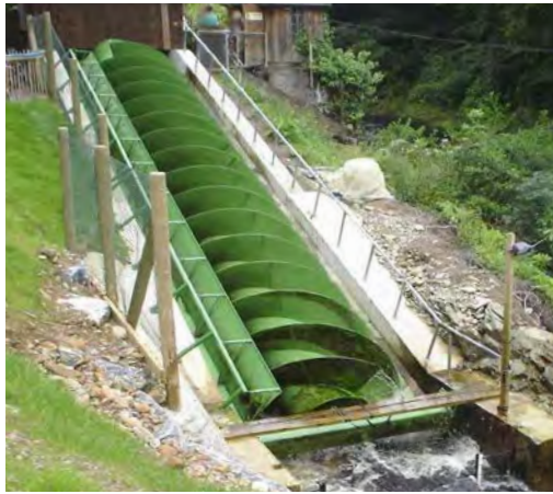
Source: The New England Hydropower Company Figure 1-8. Archimedes screw for hydropower generation
