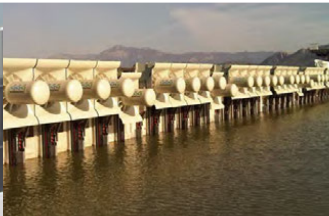
Source: Andritz Hydro Figure 1-10. Modular application of standard turbine runners to an existing dam
