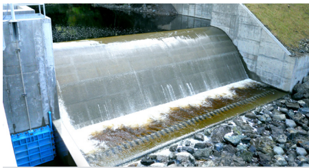
Young's Creek Hydro Project in Washington State, 2011 (7.5 megawatts) Photo credit: Snohomish County Public Utility District
