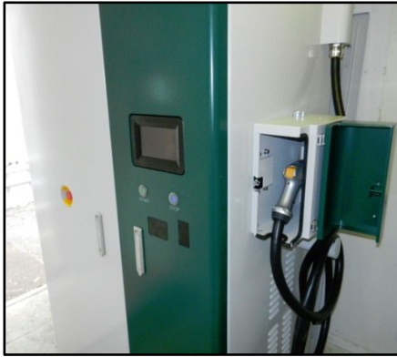
Figure II-19: VLI-EV DCFC unit installed at the EZ Messenger fleet location with both CHAdeMO and combined charging system connectors (the CHAdeMO connector is shown).
