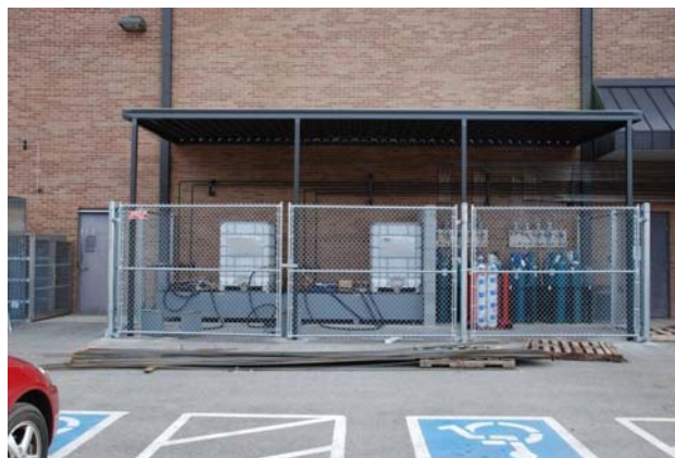
Figure 2. Photograph showing fuel tanks (left) and the calibration gas racks (right) used for engine and cell operation.
