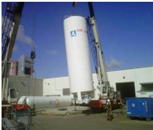
Figure II - 67: Process Gas Insulation.
