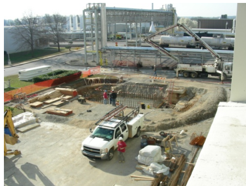
Figure II - 72: FutureFuel – Loading Dock Foundation.
