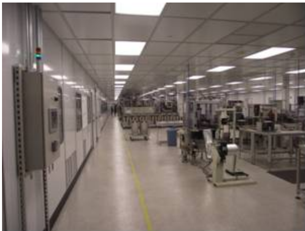
Figure II - 36: EnerDel Lithium-ion Cell Production and Battery Pack Assembly – Completed Dry-room – Hague Rd.
