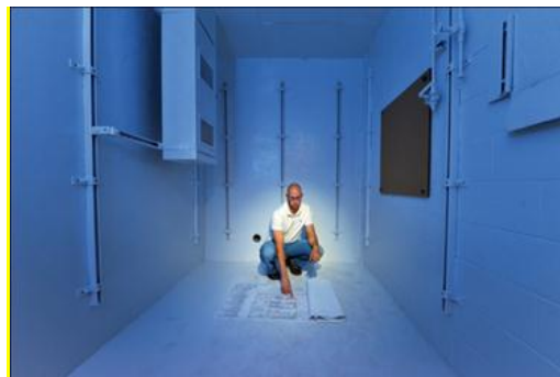
Figure II - 122: Completed renovated test cell in the abuse facility.
