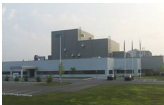
Figure II - 57: Toda America Inc. Battle Creek Facility, Phase 1.
