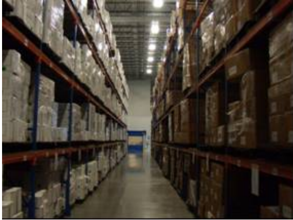
Figure II - 50: Completed warehouse (Phase 1 Project in Charlotte, N.C.)
