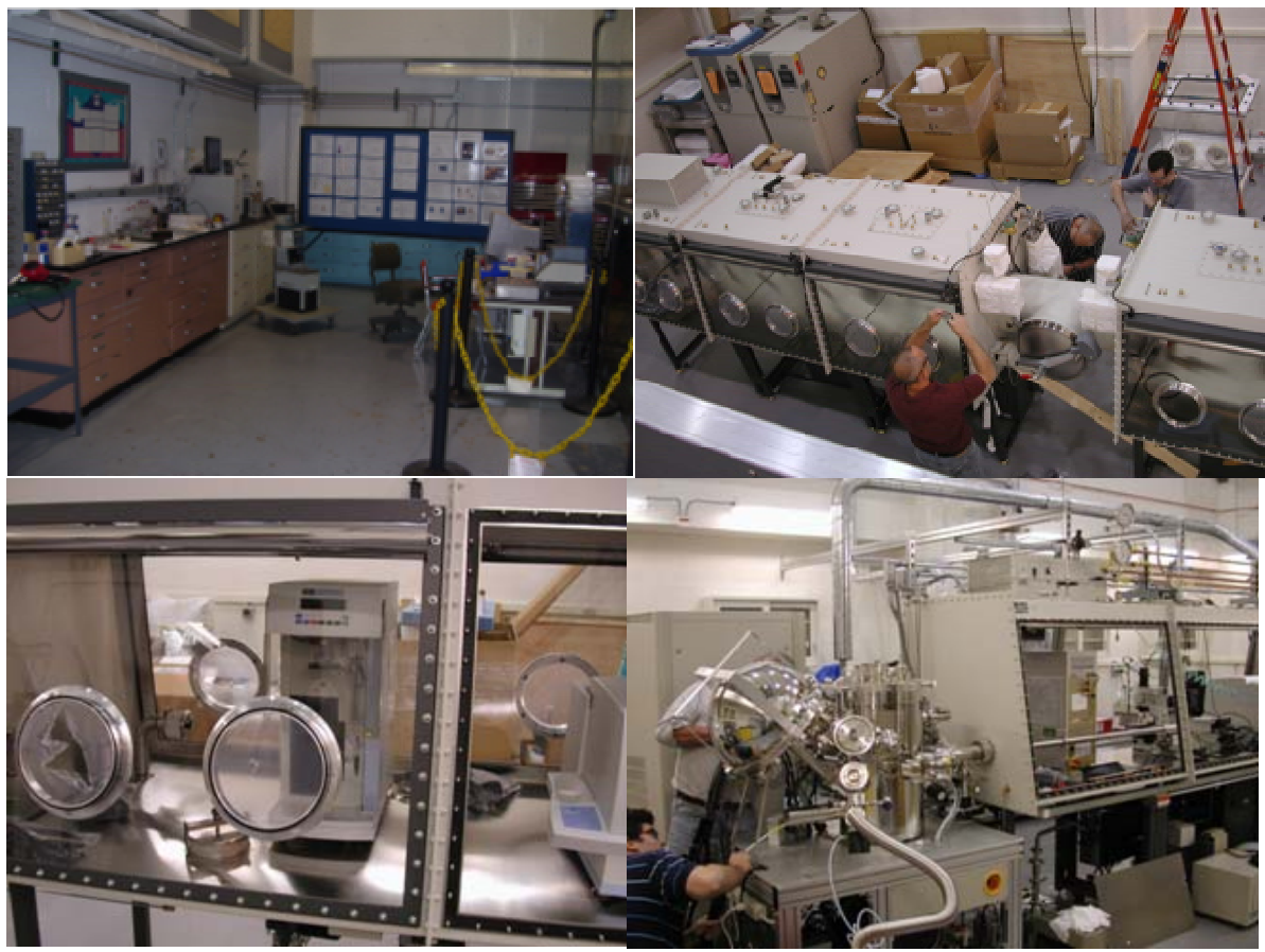
Figure II - 108: Photographs showing progress in modifying the laboratory space. Clockwise, from the upper left: starting condition; installing glove box in facility after renovation; installing the thermogravimetric analyzer in glove box; and attaching the XPS unit to the glove box.
