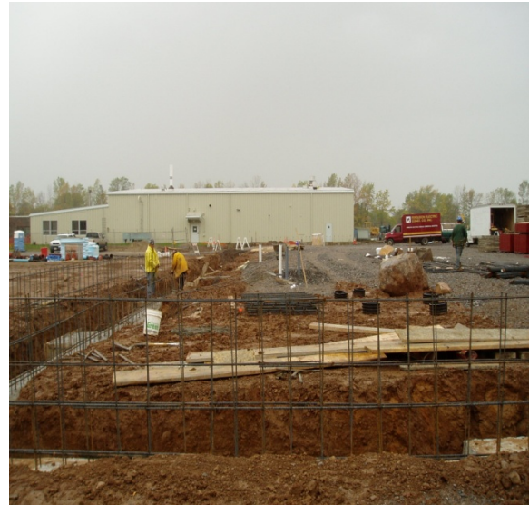
Figure II - 82: Pyrotek Production Facility Project – Construction.
