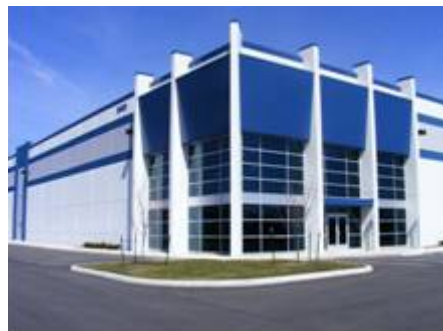
Figure II - 33: EnerDel Lithium-ion Cell Production and Battery Pack Assembly – Mt. Comfort Facility.
