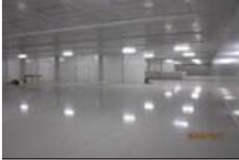
Figure II - 25: Midland, Michigan Manufacturing Facility – Dow Kokam, LLC (cont'd).
