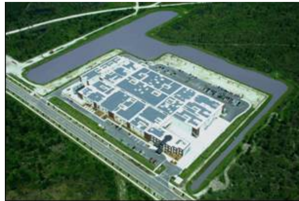
Figure II - 49: Saft Factory of the Future – completed
