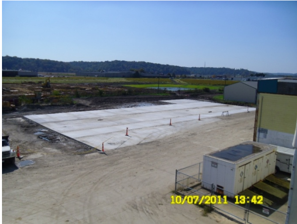
Figure II - 92: Toxco – Preliminary Building Site.
