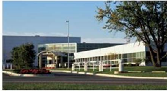
Figure II - 85: HTTP LLC, H&T, Trans-Matic Manufacturing Facility.
