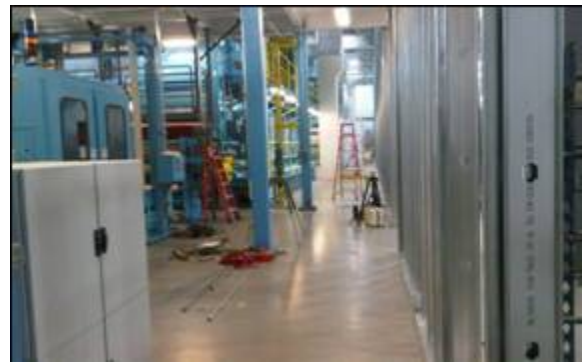
Figure II - 55: Equipment Installation Activity (Phase 2 Project in Concord, N.C.)
