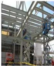
Figure II - 58: ARRA-supported Production Facility Project – Chemetall Foote Corp.
