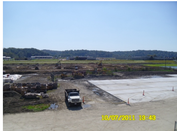
Figure II - 91: Toxco – Concrete Pad – Site Development Facilities.
