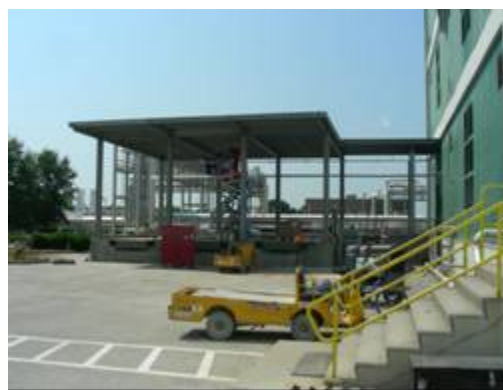
Figure II - 73: FutureFuel – Loading Dock.
