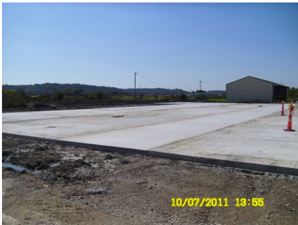
Figure II - 93: Toxco – Base Construction.
