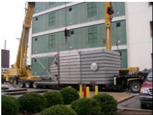
Figure II - 76: FutureFuel – Dryer Baghouse-1.
