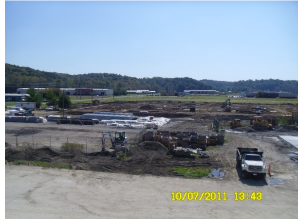
Figure II - 90: Toxco – Site Development.
