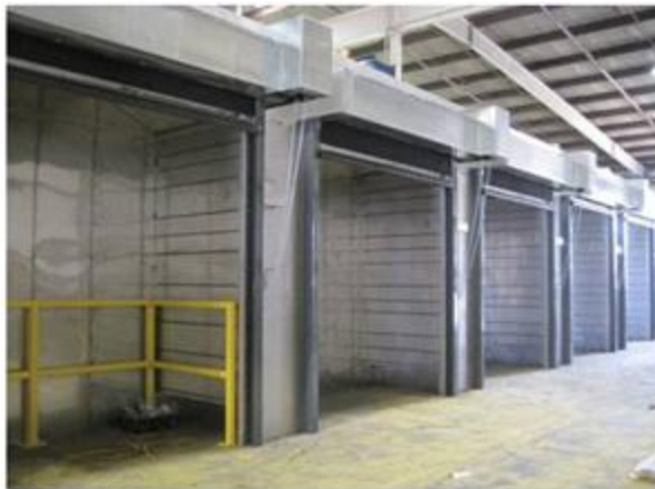
Figure II - 13: Optimized Lead Plate Curing Operation in Columbus, Georgia Exide Battery Plant.
