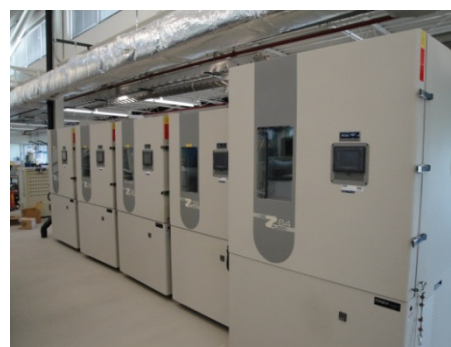
Figure II- 11: Environmental Chambers at the ARRA-sponsored NREL’s Facility
