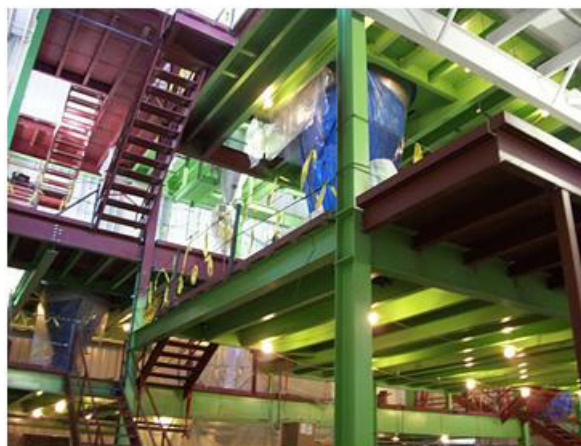
Figure II- 6: Interior construction and equipment installation in progress.
