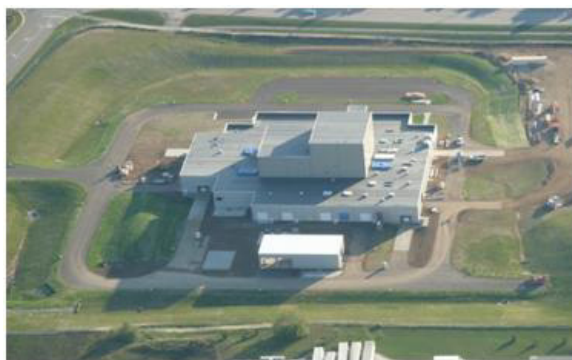
Figure II- 5: Toda America Inc. Battle Creek Facility construction in progress.
