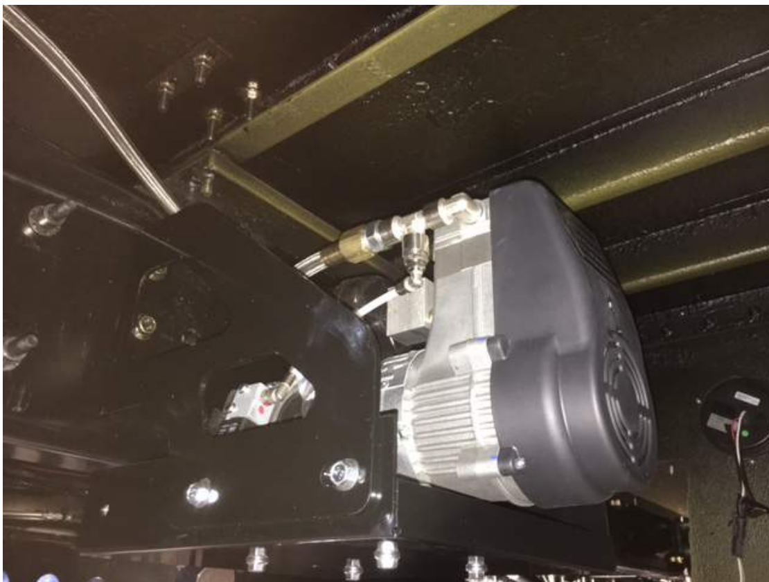
Figure II.5.2 - Air Compressor Installation in Bus P1
