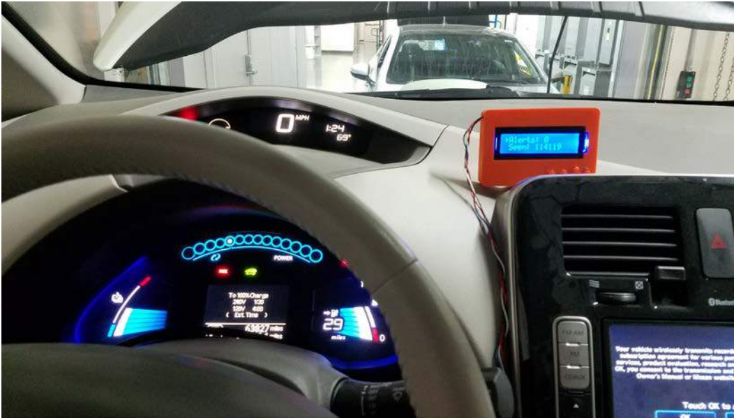
Figure IV.4.3 - DSM Installed in Nissan Leaf – Showing Status
