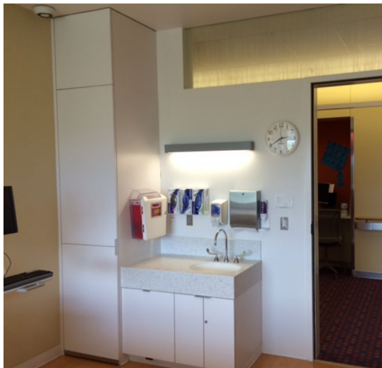
Figure A8: Hospital D patient room showing the entry area with separate sink light and push-button controller near the door.
