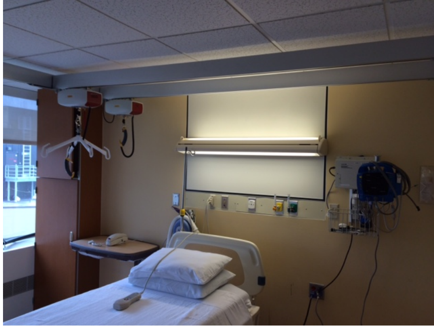
Figure A1: Hospital A patient room showing the wall-mounted luminaire at the headwall. The luminaire is hinged so that the light from the upper section (shown directed upwards here) can be directed towards the bed during an examination.
