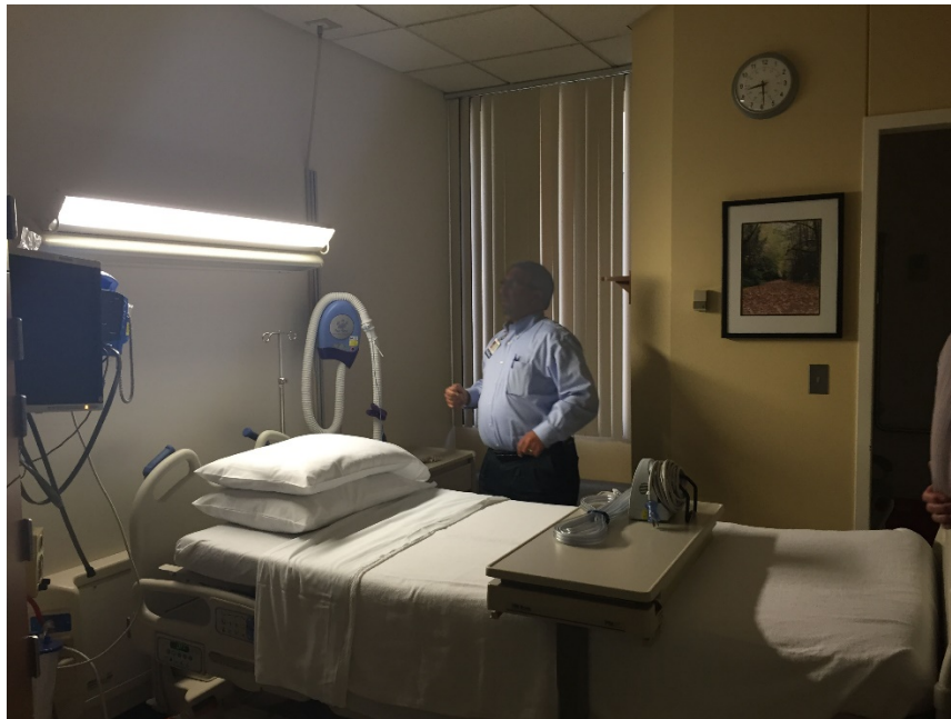
Figure A6: Hospital C patient room showing the wall-mounted luminaire with a hinged upright section. The upright section is in the examination position, directing its light toward the patient bed. The wall-mounted luminaire is the only electric lighting in the room.
