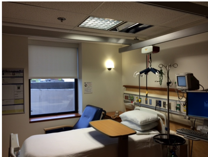
Figure A4: Hospital B patient room showing the multi-function recessed luminaire above the bed. This was the only luminaire in the rooms originally. A later upgrade added the wall sconce luminaire for the guest area, a recessed downlight in the doorway entry area, and a step-light-style nightlight recessed into the wall.
