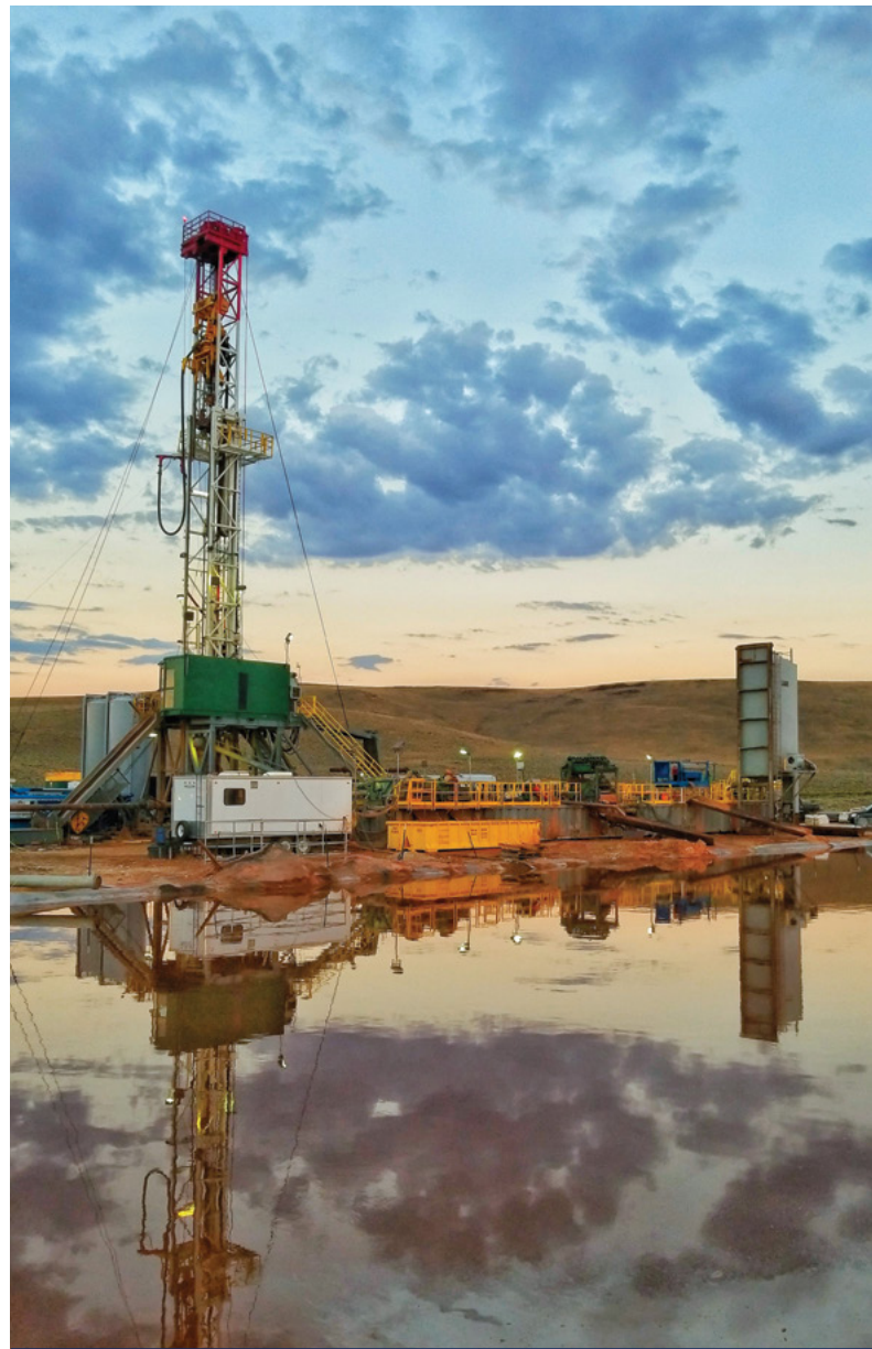
Drilling a geothermal well at twilight at McGuinness Hills, Nevada.
