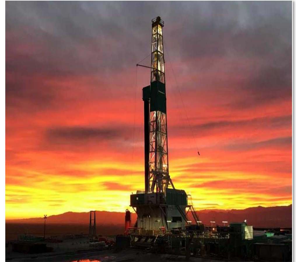
Shown here is a drilling rig at the FORGE site outside of Milford, Utah. RD&D at FORGE continues through 2024 and will drive technological advances in enhanced geothermal systems. Photo: Eric Larson / FORGE Utah
