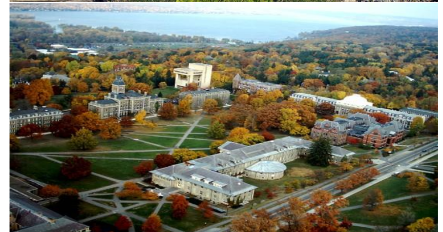
Military installations and university campuses are among the variety of locations that can benefit from direct use geothermal. Shown here are the Hawthorne Army Depot in Nevada and Cornell University in New York.
