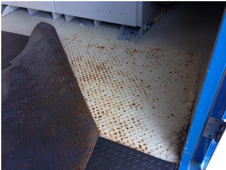
Figure 60: Generator room floor corrosion due to continual presence of mats. Mats were subsequently removed and the floor was re-painted with more robust paint.
