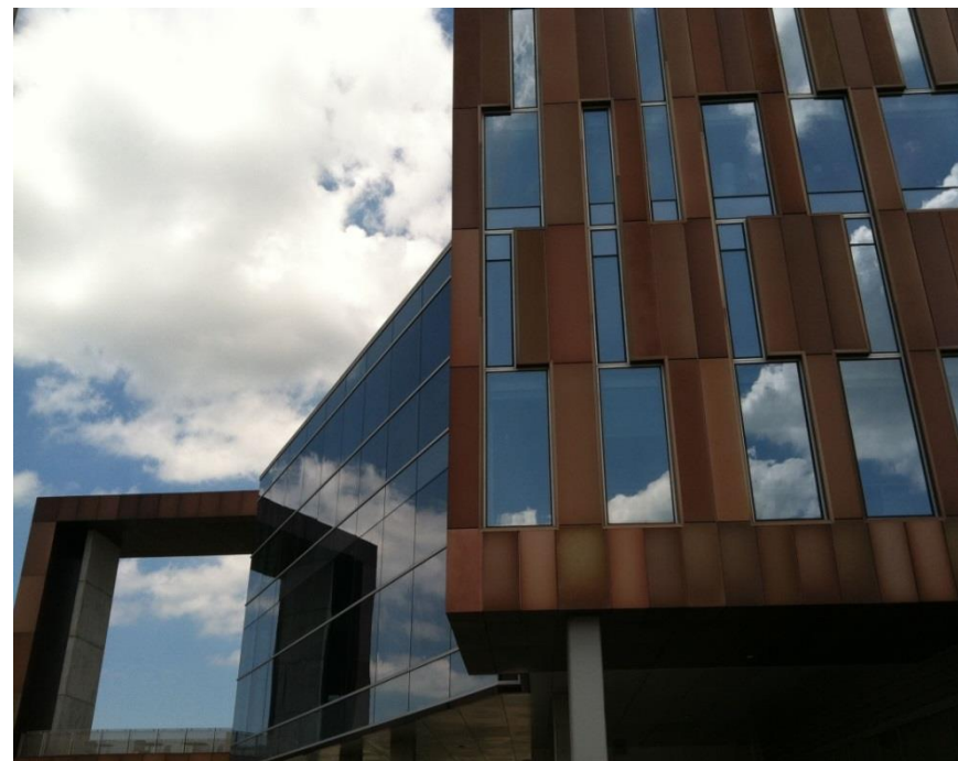
ANL's New Energy Science Building
