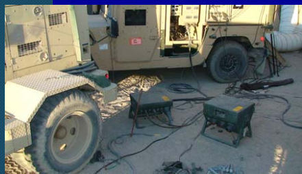
Take Almost Any Generator
