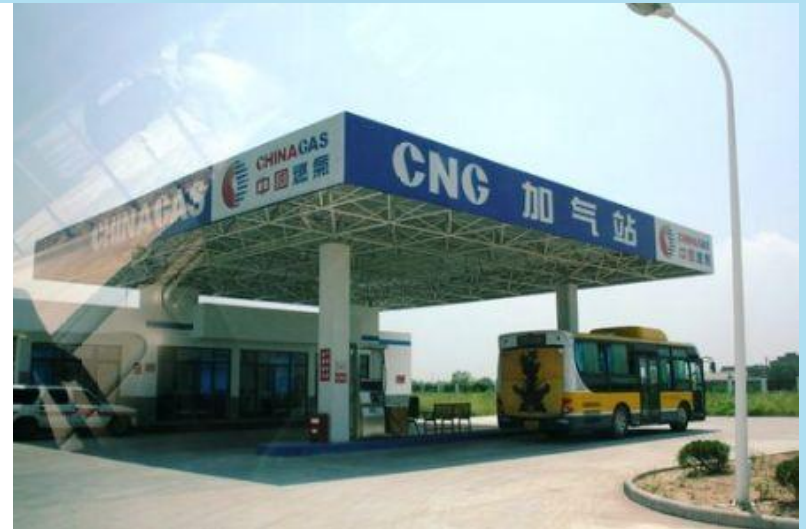
CNG refueling station
