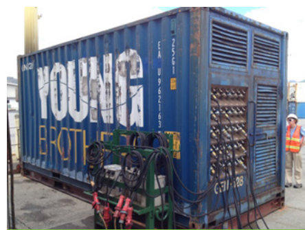
Fuel cell power generator for maritime refrigeration.
